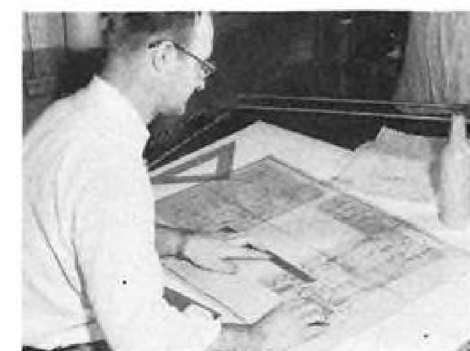
Big head start. Kodalith Film prints of elements which are repeated from time to time are kept on file. When a new design calls for any of these elements, the draftsman merely tapes the right films on clear acetate and orders an Autopositive. No redrafting!
