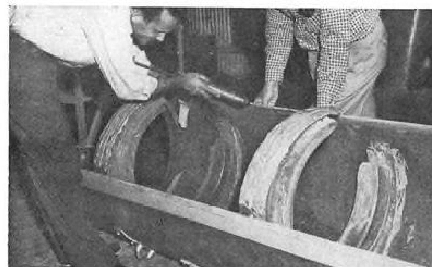
3. SKIN EDGE is coated with adhesive for mating section.
