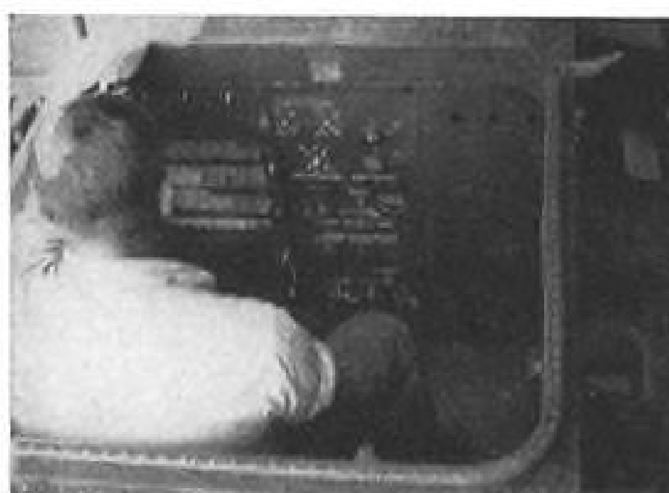
COCKPIT OF BEACH CRADLE has controls for land steering. Operator coordinates maneuvers with plane's pilot via radio.
