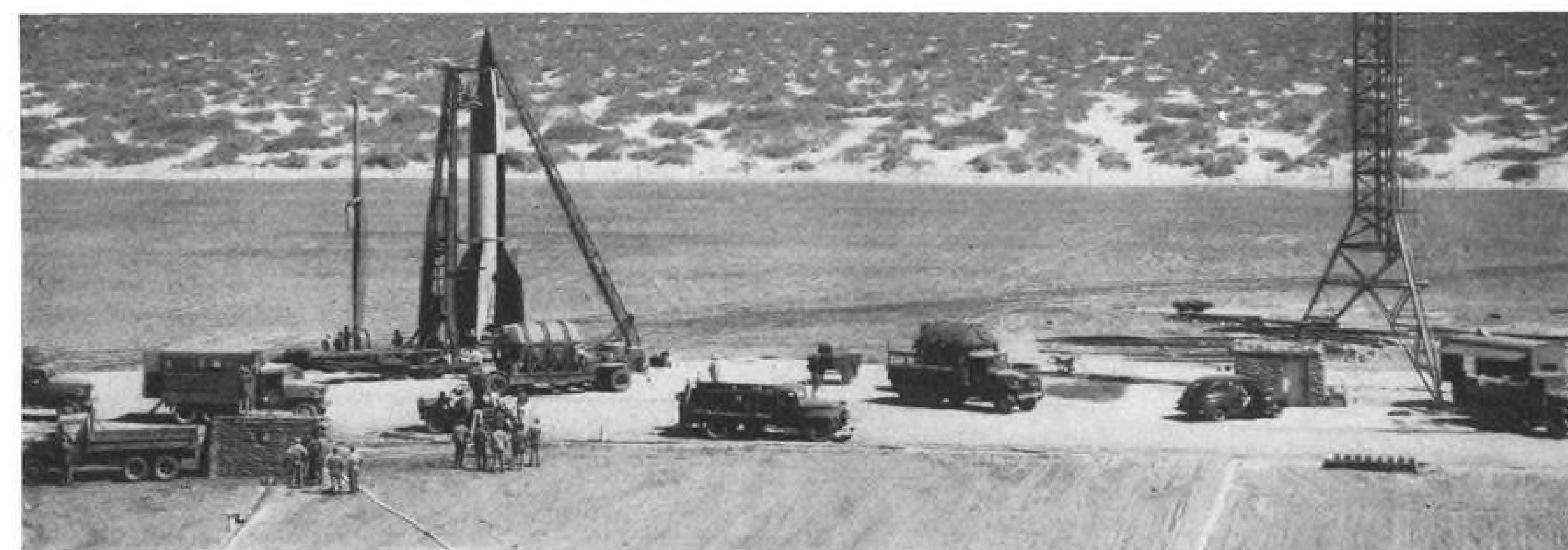
V-2 VEHICLES are portion of the mobile fleet required to transport, erect, service and launch this early ballistic missile.
