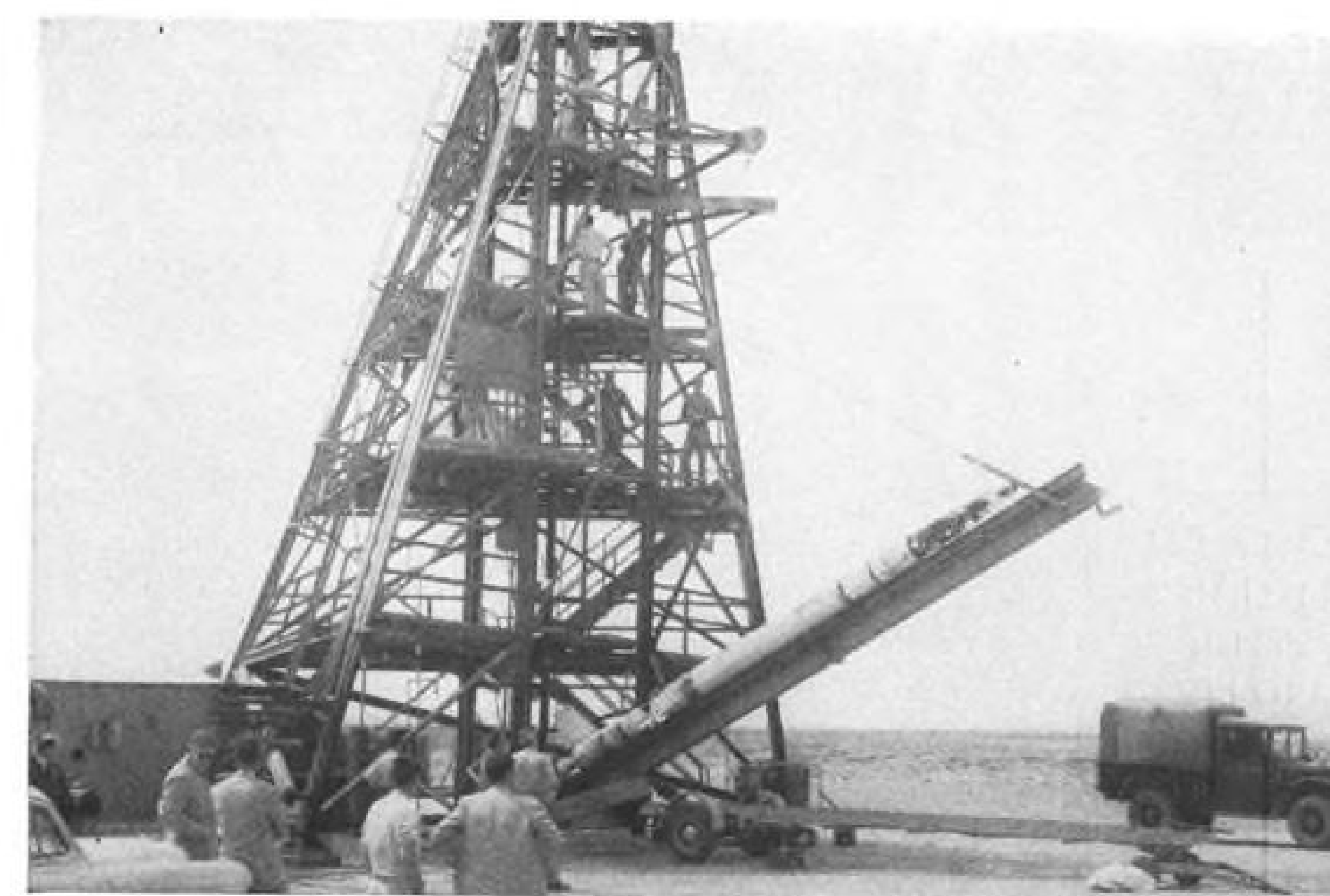
HIGH-ALTITUDE ROCKET is raised on its cradle to launching tower, prior to first flight.
