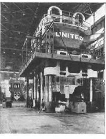
50,000-ton press (background) and 35,000-ton press are housed in 10-story, 12-acre building adjacent to Alcoa's forging and casting works in Cleveland.
