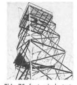
This 75 foot winch test tower is capable of simulat ing flight conditions and loads up to 30,000 lbs.
