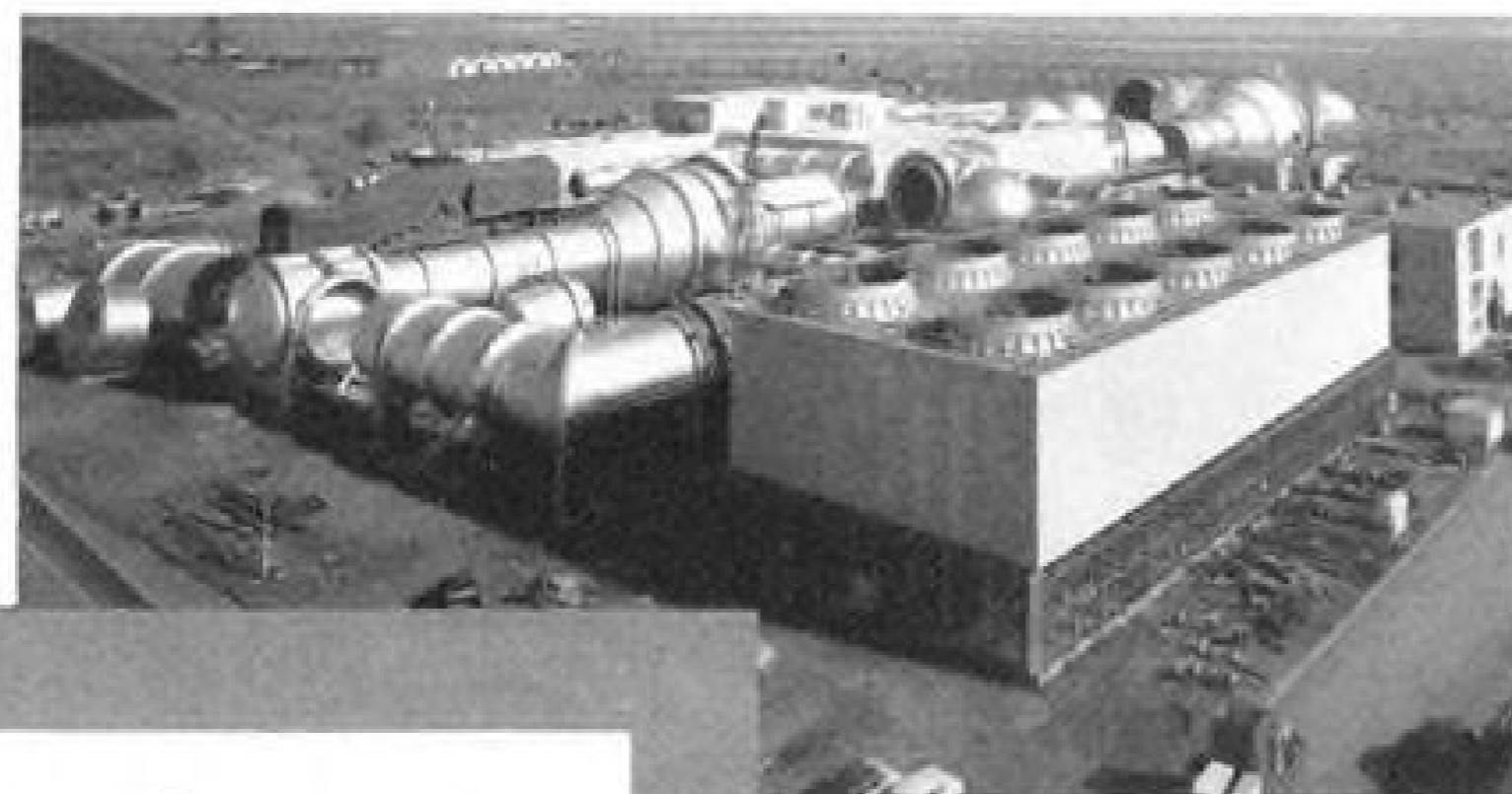
Below: Supersonic wind tunnel located at Ames Aeronautical Laboratory, operated by the NACA at Moffett Field, Cal. All tunnel sections except valves and throat fabricated and erected by Chicago Bridge & Iron Company.
