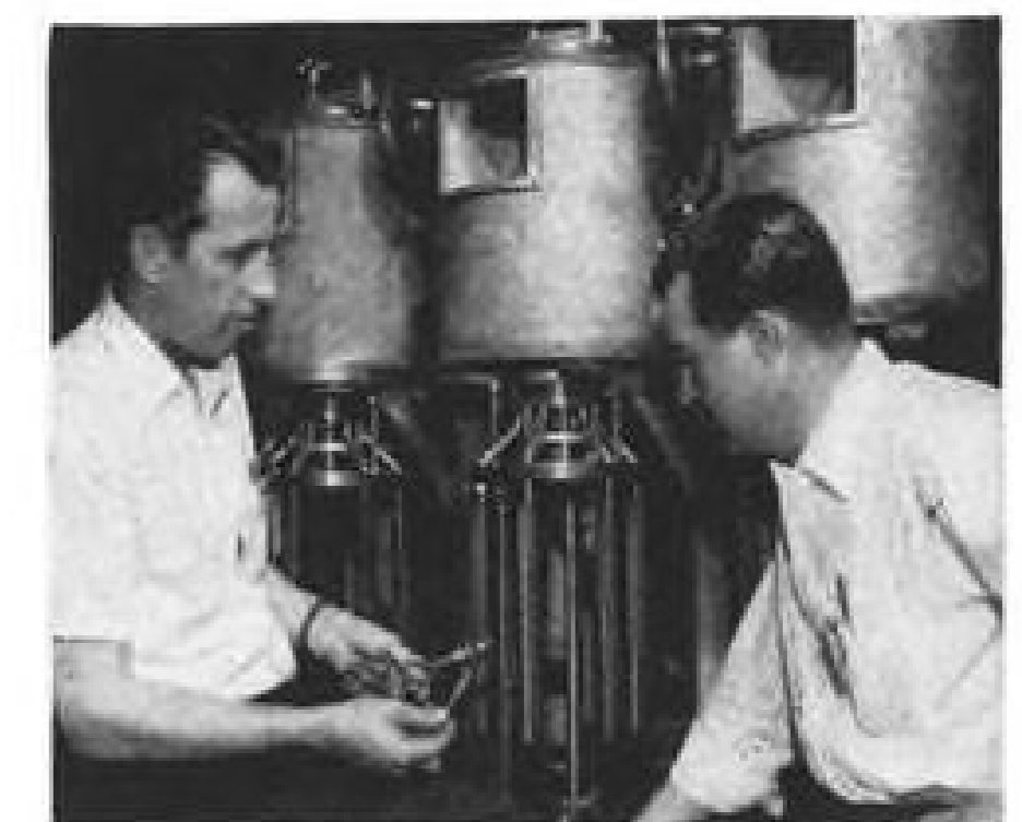
These two development engineers are evaluating a new fuel nozzle. The equipment in the background is designed to test the performance of fuel systems.
