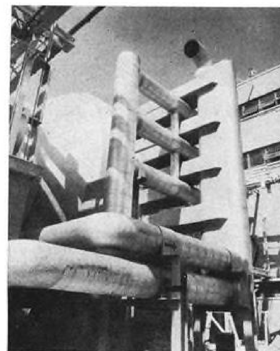
LARGE-SIZE refrigeration piping leads to intercooler (left) and test wing (right).
