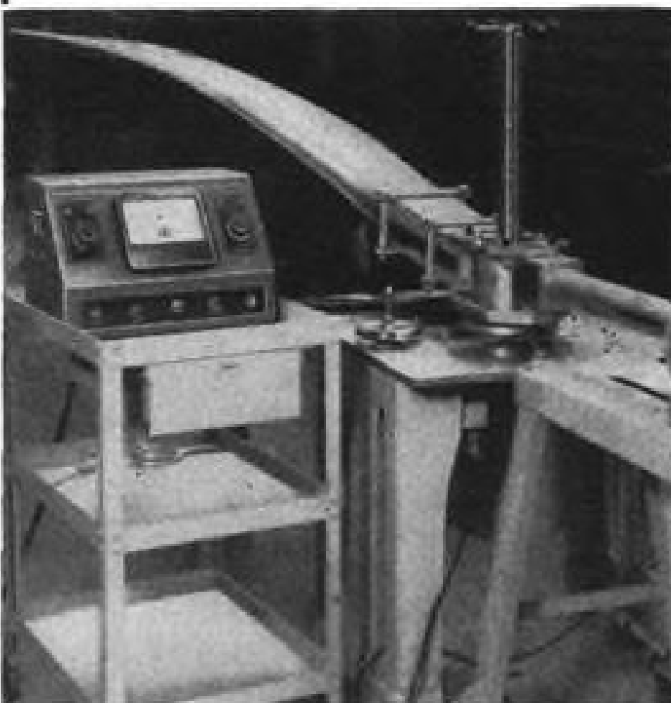
Kaman Aircraft Corp. Now Balances Their Helicopter Rotor Blades And Assemblies On a Dean And Benson Machine
