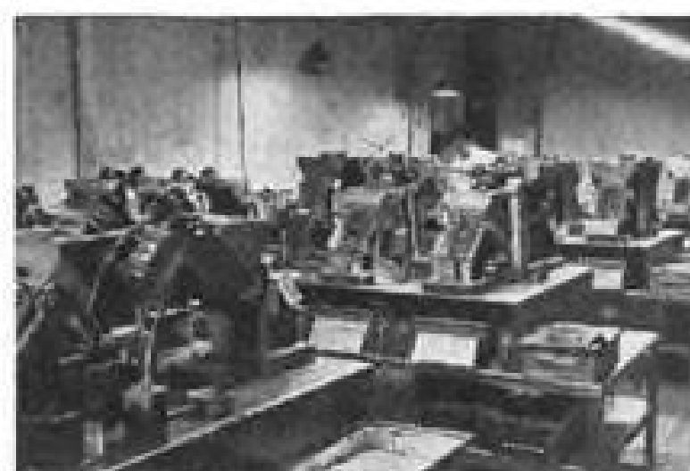
These gauges sort balls into lots according to required diameter limits.
