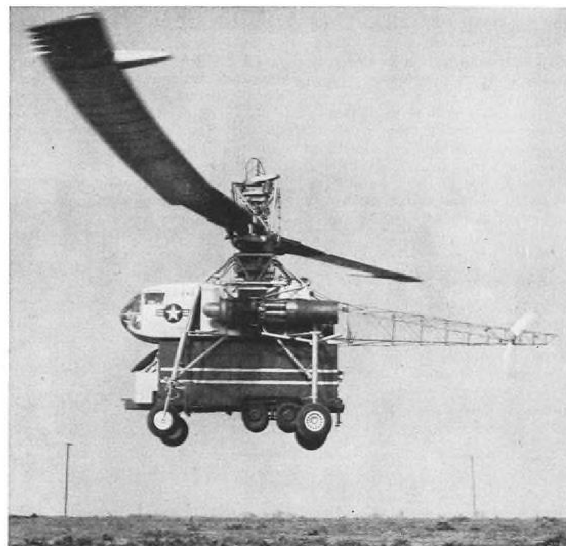
. . . AND THE WORLD'S LARGEST HELICOPTER picks up its record load and flies away. Hughes officials say helicopters of the same design could carry 10-ton loads, including tanks.
