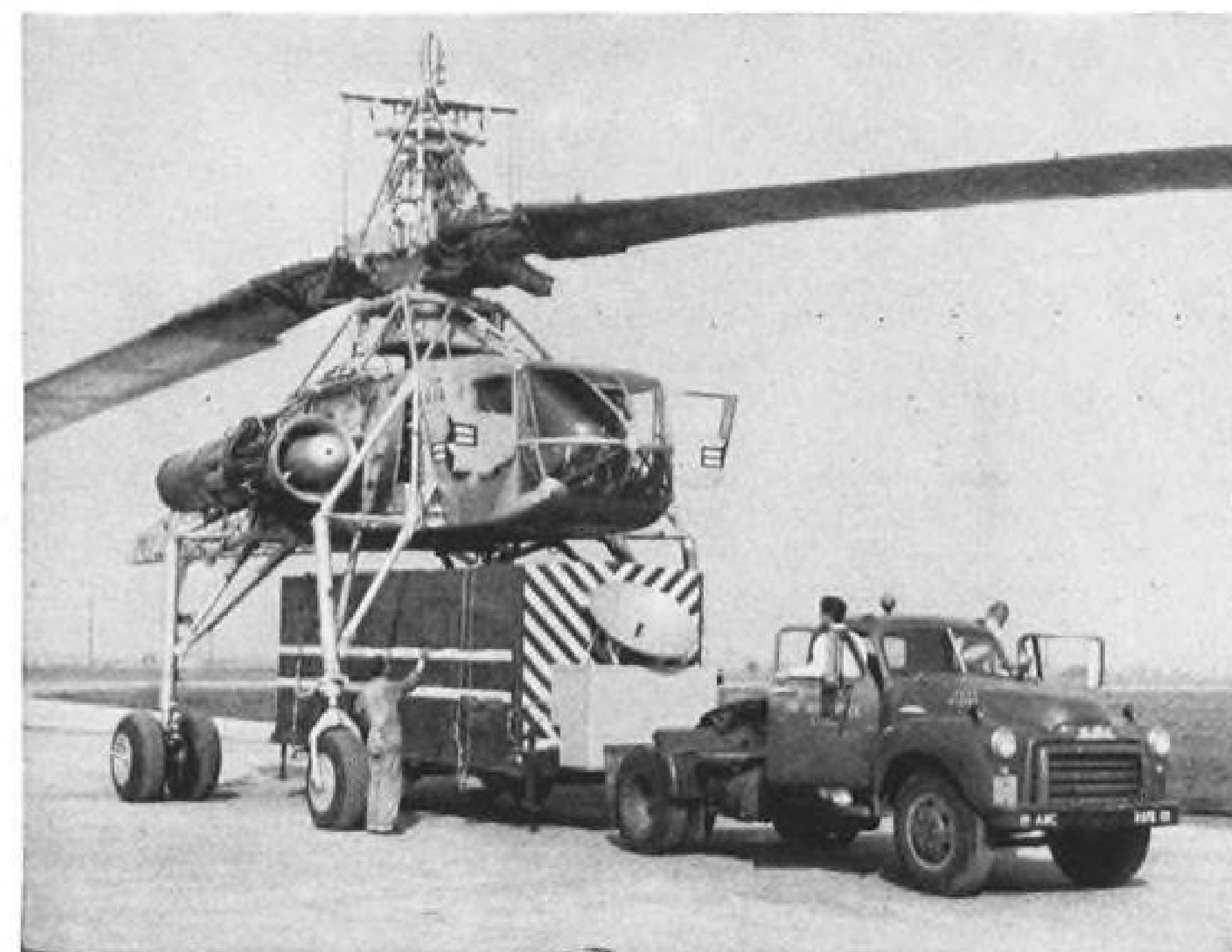
JET POWERED XH-17 developed by the Aircraft Division of Hughes Tool Co. gets ready above to airlift a USAF trailer van, largest object ever to be carried by a helicopter. Truck pushes the van into position between the XH-17's stilt-like legs . . .
