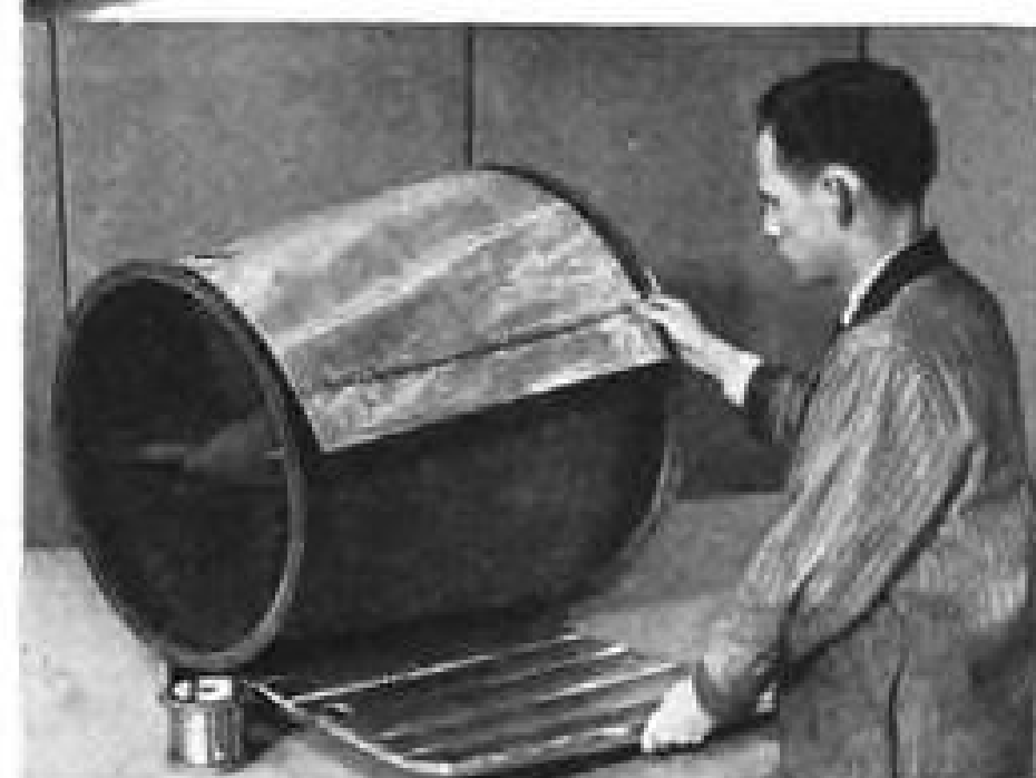
Thermoflex Thermal Insulation Blanket being applied to a jet engine exhaust cone. Special grooving assures precision fit around cylindrical and conical surfaces... allows for expansion at high temperature.
