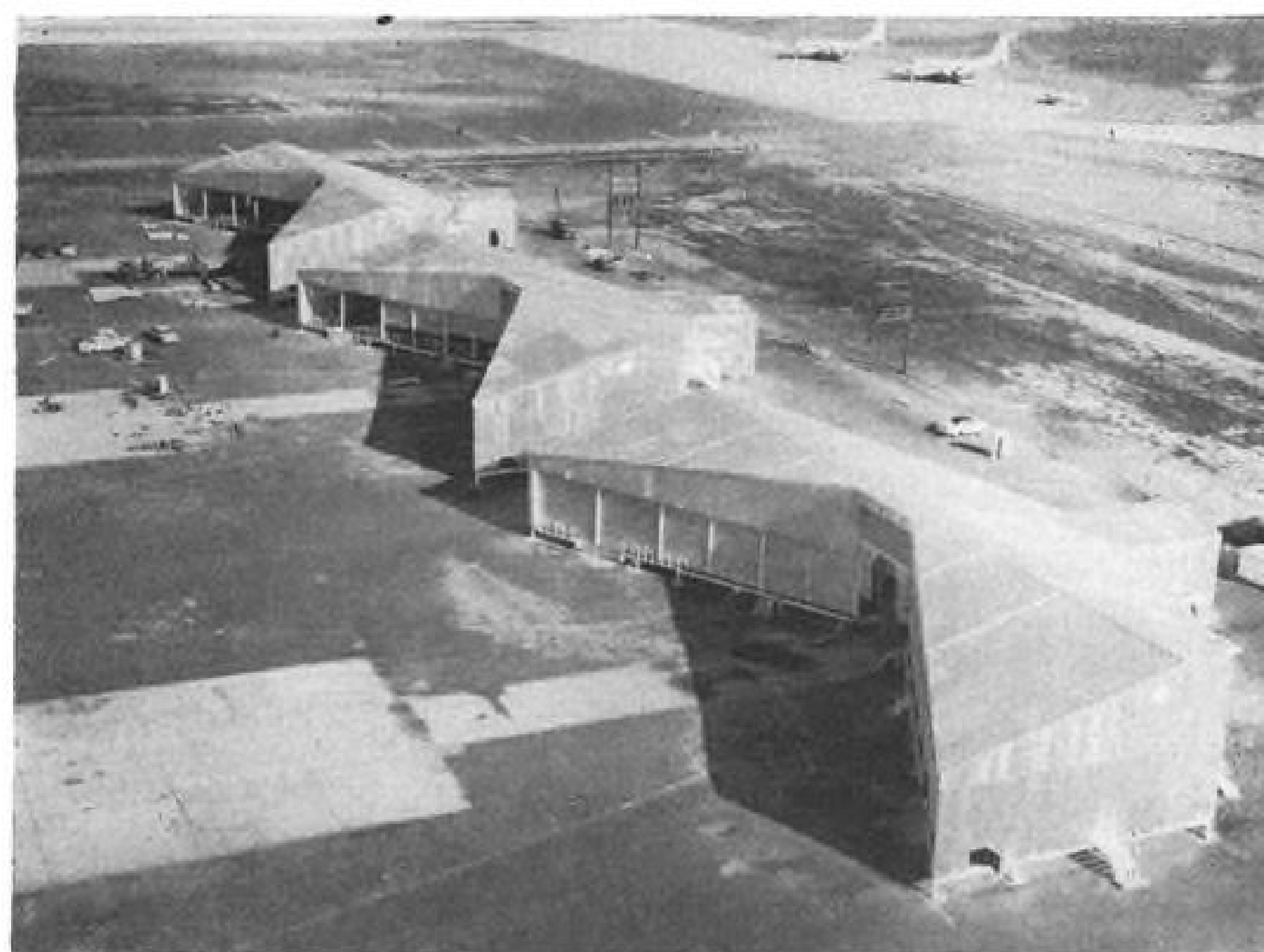
THESE NOSE DOCKS can be disassembled for air transport, cost $170,000 each.
