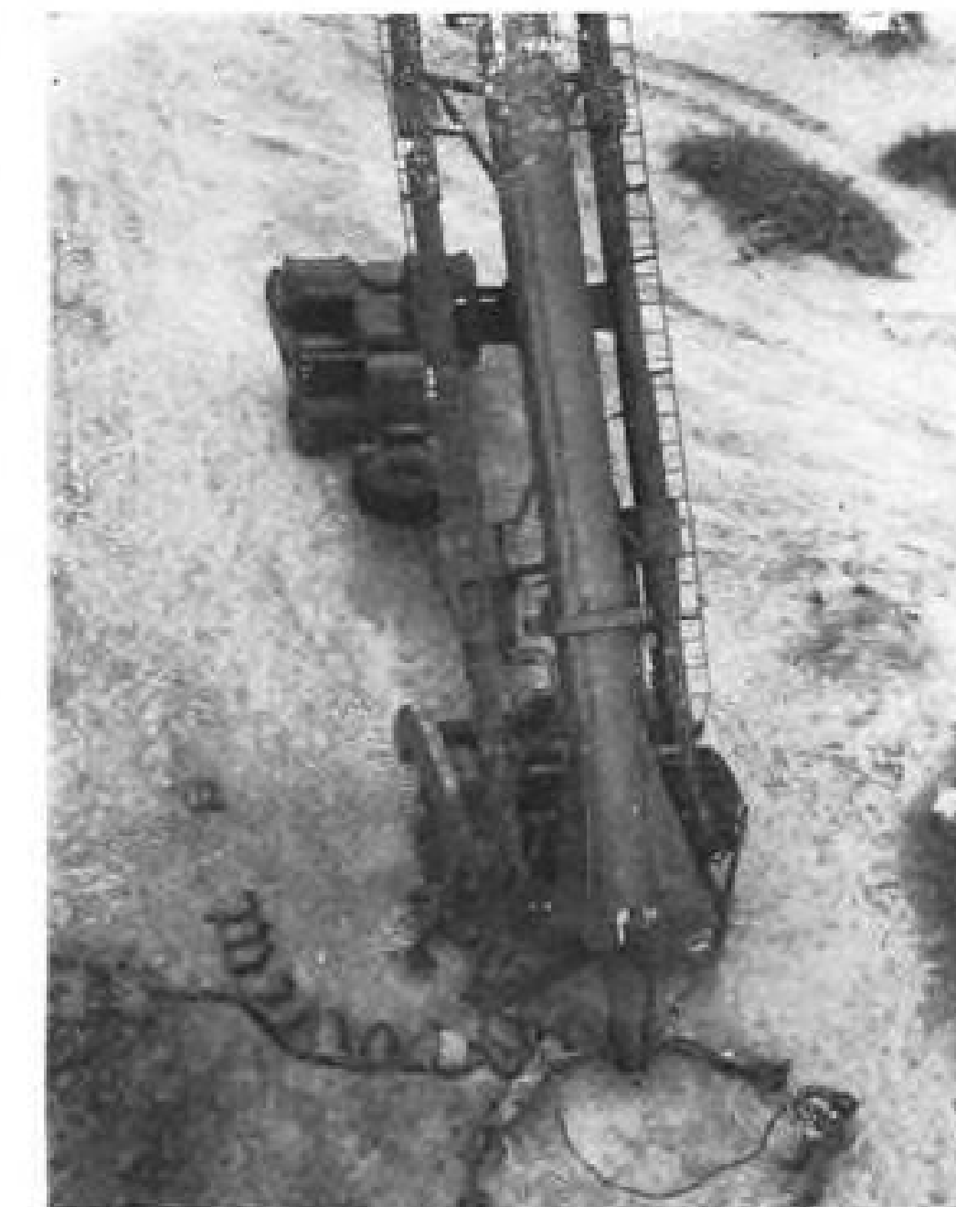
MEMBER of battalion using remote control box to erect Corporal on launcher.
