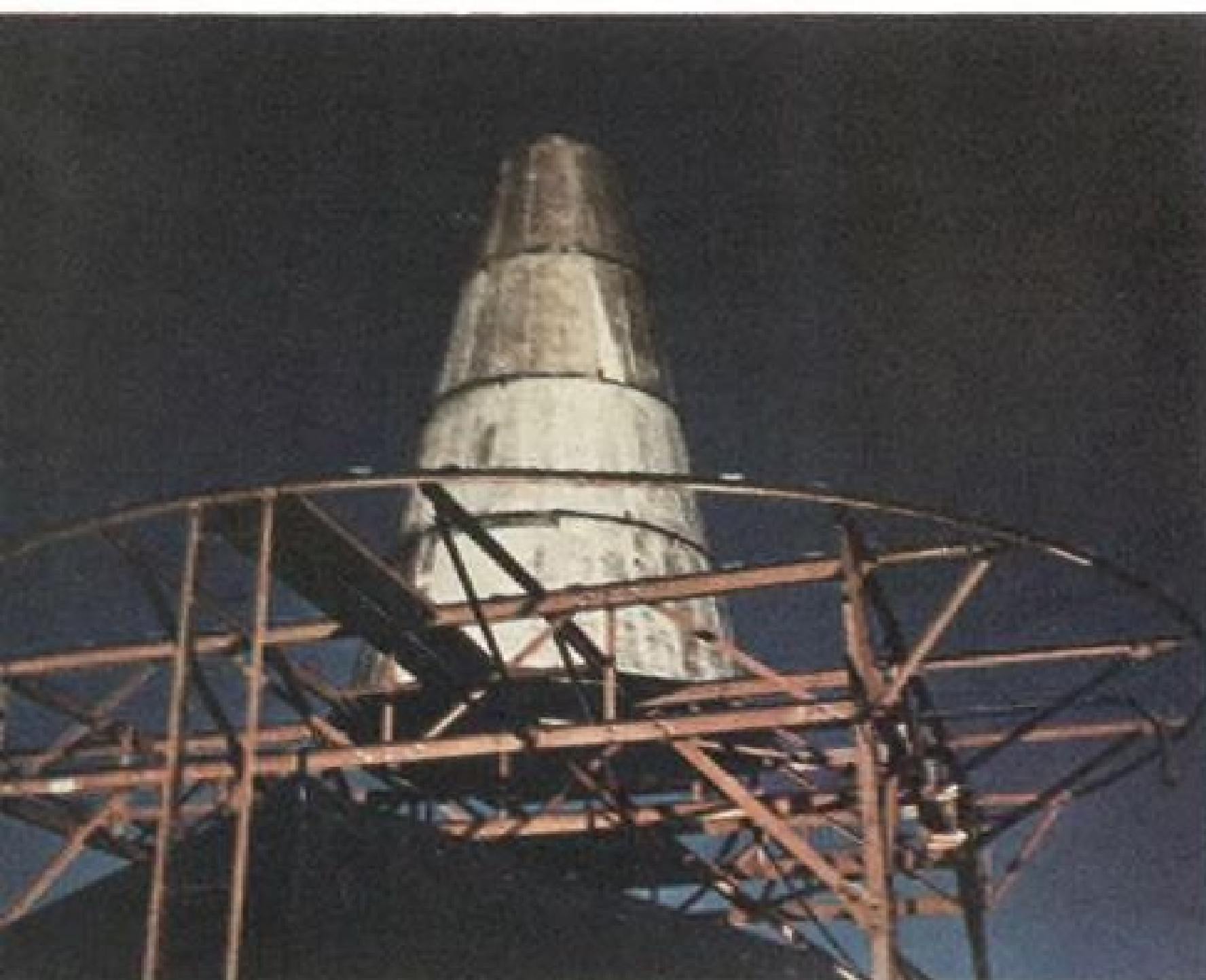
ANTENNA at Rome ADC permits co-location of TACAN, VOR
