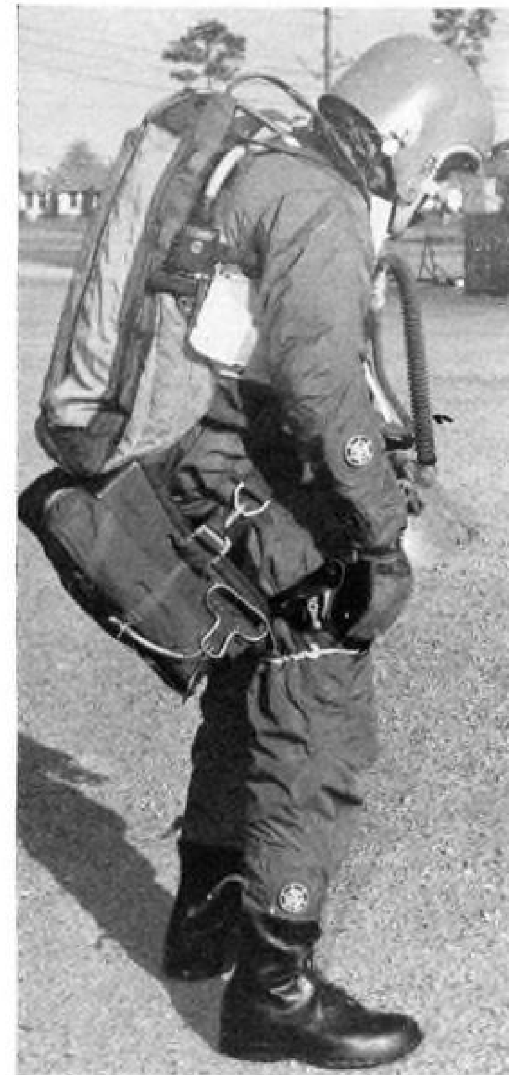
DRESSED TO LEAP from a balloon 18 miles above the earth, Capt. Henry Neilsen bows under the weight of five shells of protective clothing comprising an artificial environment, oxygen and other survival gear.
