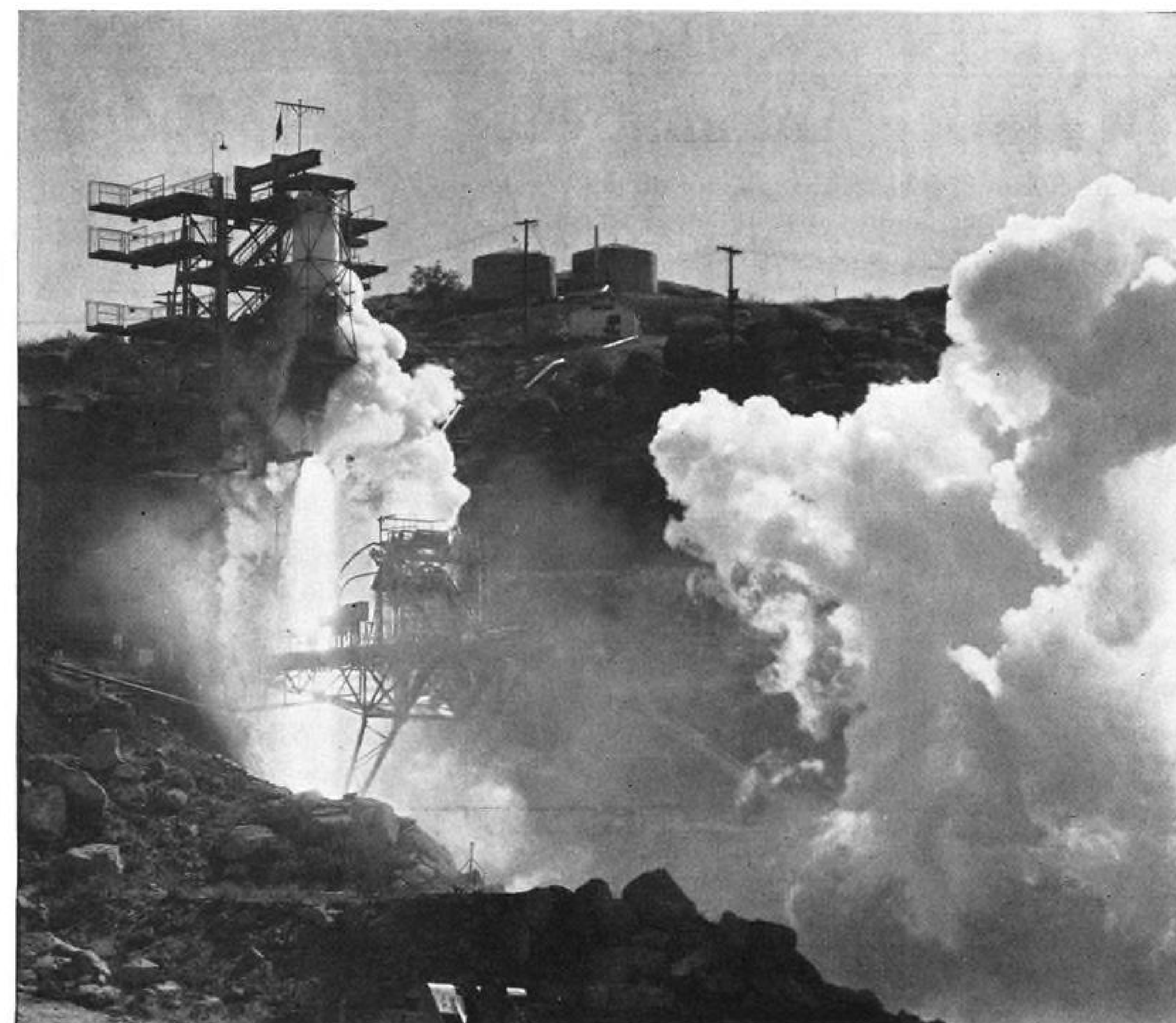
Actual test firing of a modern ROCKETDYNE rocket engine at the Field Test Laboratory in the Santa Susana Mountains.
