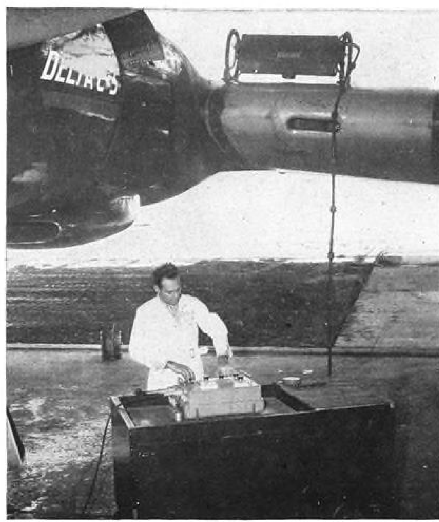
RADIOGRAPHIC SERVICE being performed (left) at Idlewild Airport by Burgoyne X-ray and Metal Testing Laboratories, Inc., of a wing. Radiographer positions film inside wing. Andrex X-ray New Cassel, L. I., on Constellation belonging to major airline. equipment (right) in typical set-up for X-raying wing spar.
