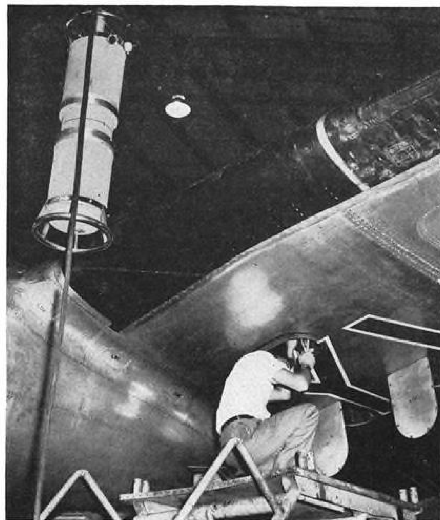
RADIOGRAPHIC SERVICE being performed (left) at Idlewild Airport by Burgoyne X-ray and Metal Testing Laboratories, Inc., of a wing. Radiographer positions film inside wing. Andrex X-ray New Cassel, L. I., on Constellation belonging to major airline. equipment (right) in typical set-up for X-raying wing spar.
