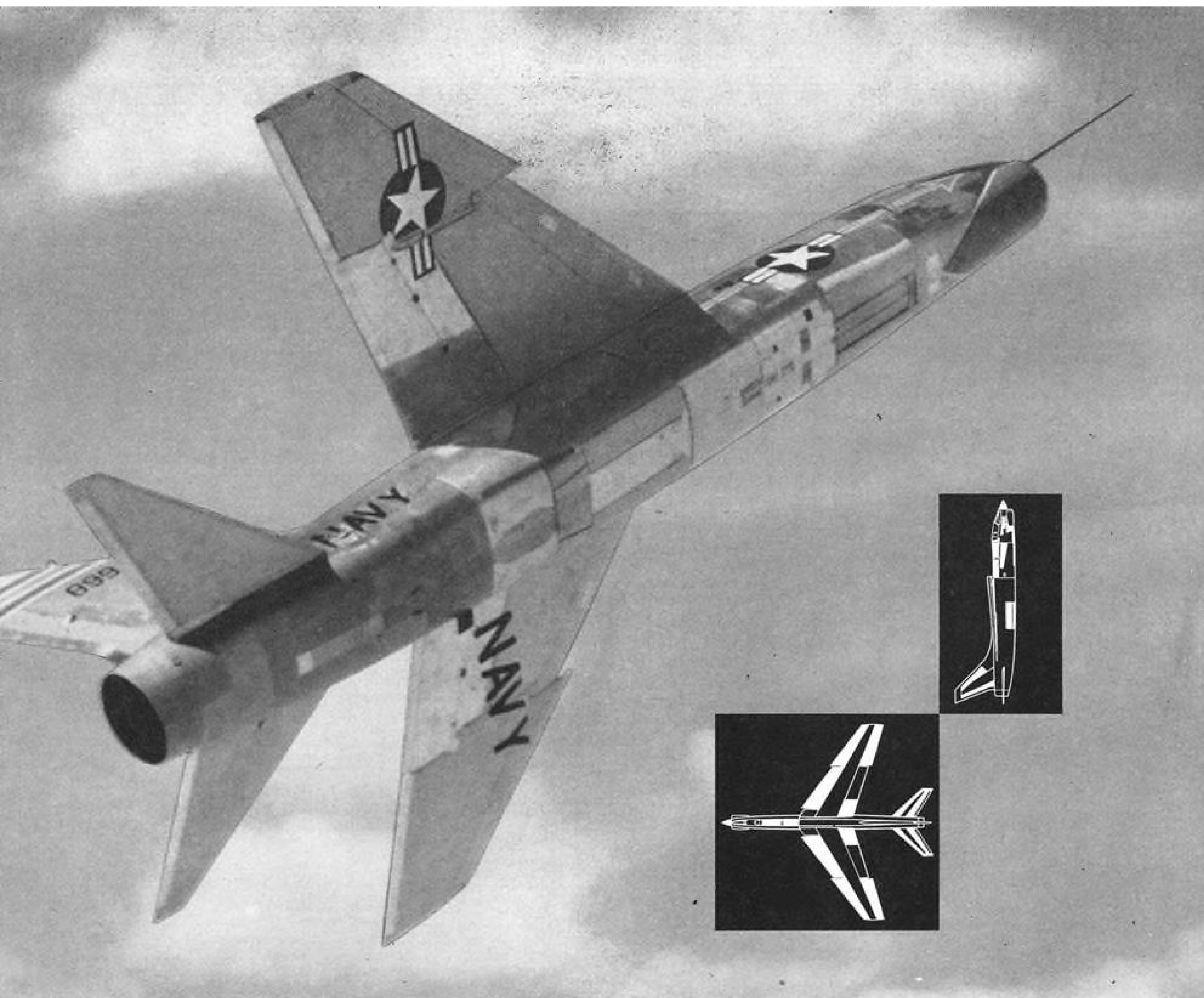
Weight-saving magnesium sheet (white areas) is used for leading edges, empennage, wheel doors and many other parts of F8U-1 Crusader.
