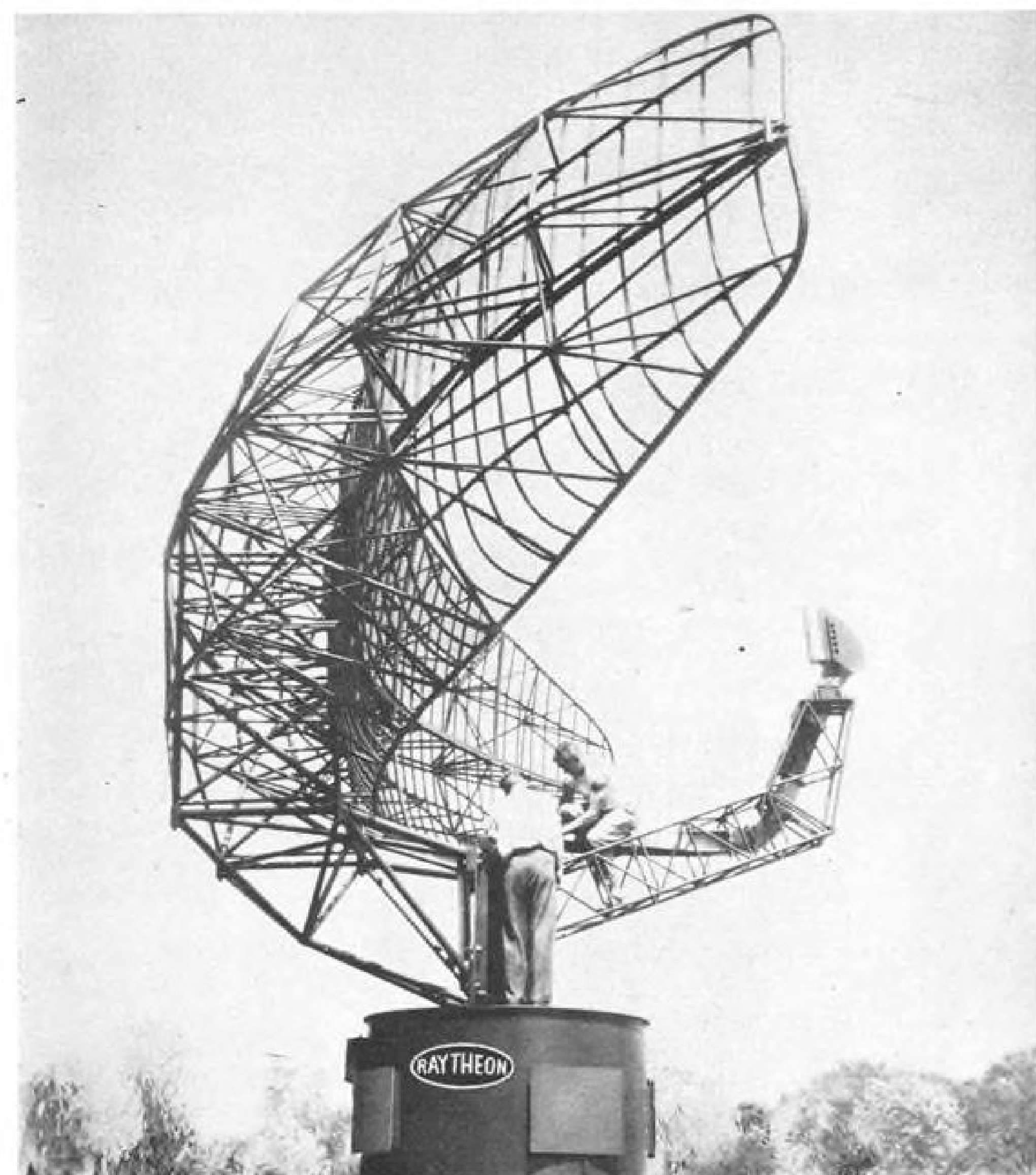
LONG-RANGE radars ordered by CAA will be installed at major airports shown (heavy circles) within two years. These will be supplemented by military radars not shown. Forty-foot antenna (below) will be used in new L-band radars to be produced by Raytheon.
