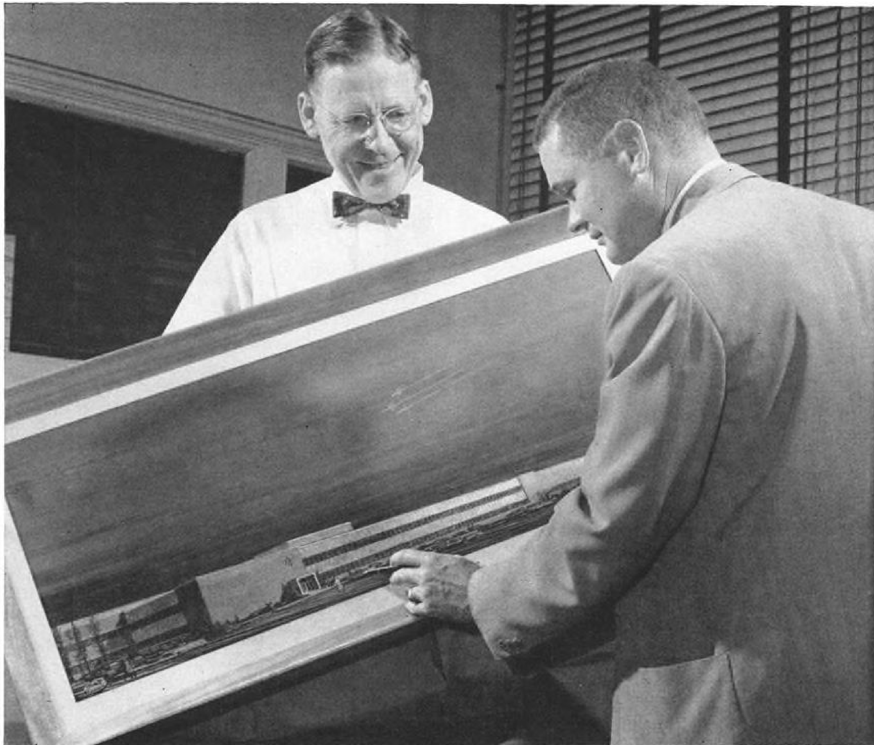
This modern, air-conditioned building is now being erected to house the Columbus Engineering Department.
