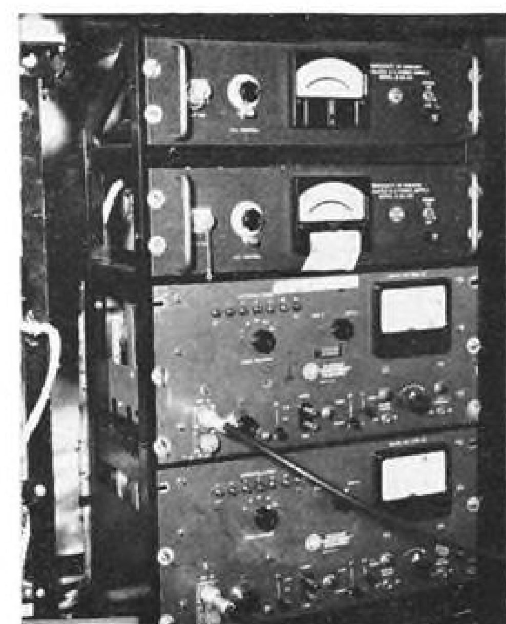
BLACK BOXES count neutrons freed in pile by cosmic particles. Upper two are scalars. Lower two are amplifiers.
