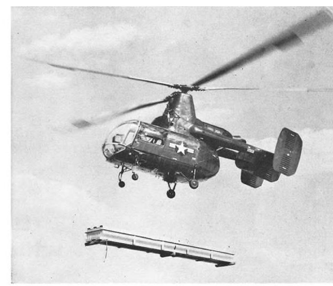
EXTERNAL cargo hook can handle loads too awkward to stow in K-600-3 cabin via clamshell doors. The K-600-3 is a modified version of Kaman's HOK-1, built for Navy.
