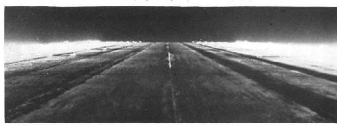
THIRD SYSTEM consists of fluorescent tubes with high output along runway edge. Light reflects on painted strips, but is better on black surface than white concrete.
