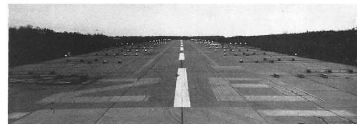
ONE SYSTEM of runway landing lights under test by CAA has bars spaced 30 ft. from runway centerline. In operational use, lights would be set flush in runway.
