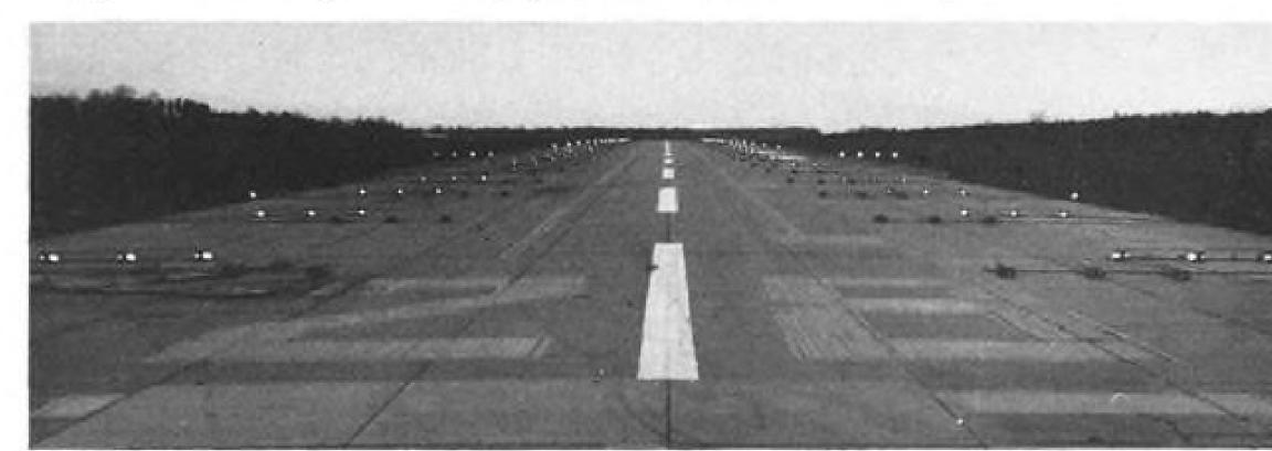
SECOND SYSTEM is similar except that the bars are spaced 45 ft. from runway centerline. Produced by Sylvania, the Elfaka runway lights originally were developed by Dutch.
