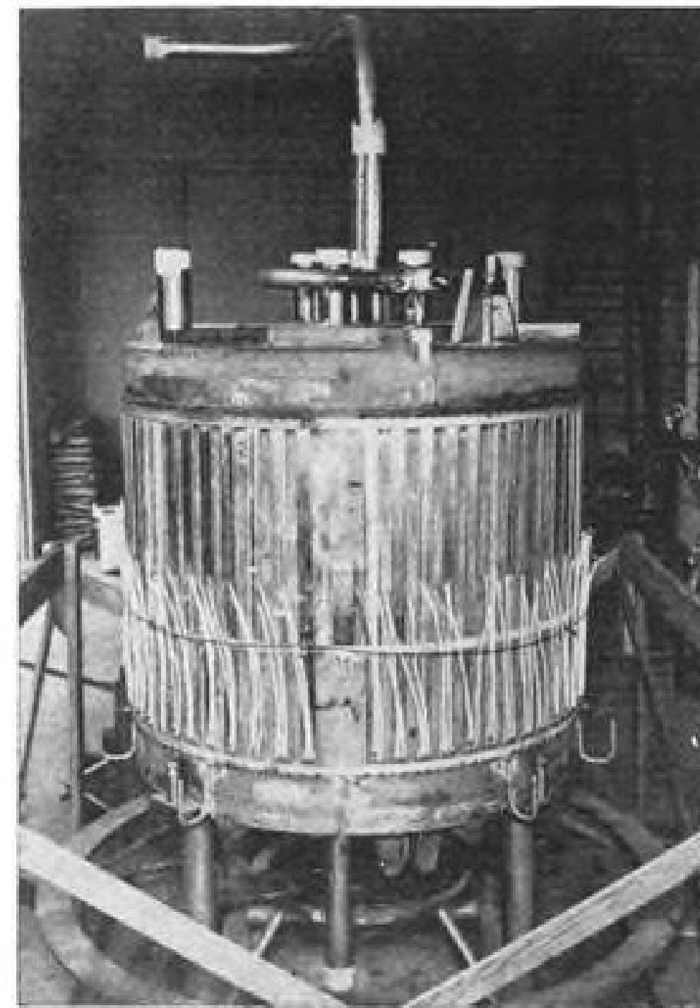
AIRCRAFT POWERPLANT reactor from experiment 21 years ago (AW May 27, p. 27). Large tube at top of 33 in. diameter reactor outlet (left) is for the sodium heat removal circuit while smaller extensions at outer rim probably provide access for flux measuring instrumentation to evaluate fission. The other pipes in the center are for regulating and control rods. The reactor, probably part of a joint Pratt & Whitney-Oak Ridge project, first became critical Nov. 3, 1954 when enriched uranium tetrafluoride concentrate was added to the molten fluoride salts being circulated around the power loop. Top of reactor core (right) shows the 66 tubes which circulated the molten fuel through the beryllium-oxide moderator-reflectors in serpentine loops. Six upright pipes in the center are fuel inlet tubes. The four hexagon-shaped holes around the fuel inlet pipes are for regulating and control rods, and two holes near the rim are for the neutron instrumentation.
