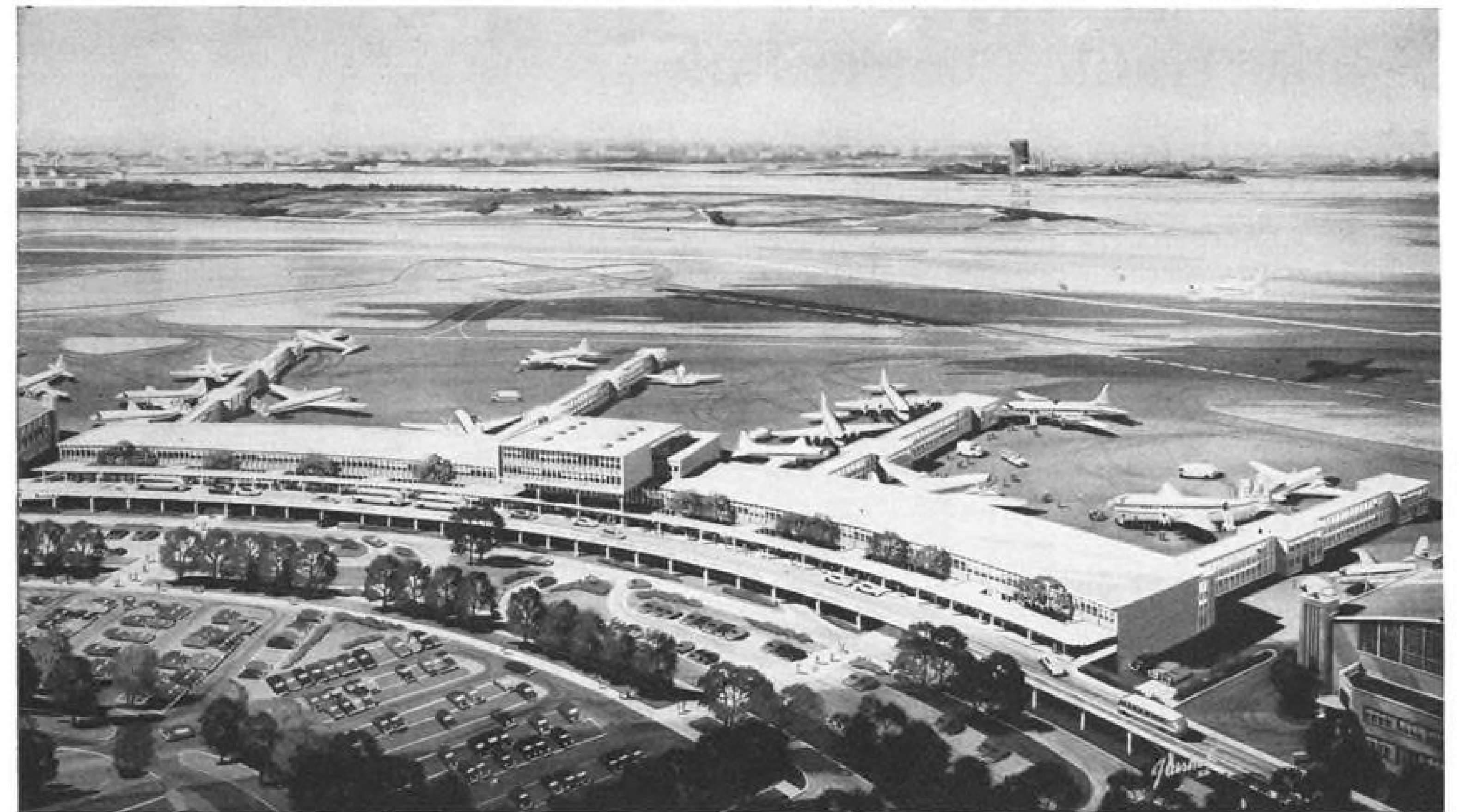
PROPOSED terminal for LaGuardia Airport features two-level passenger handling, 36 aircraft gates.
