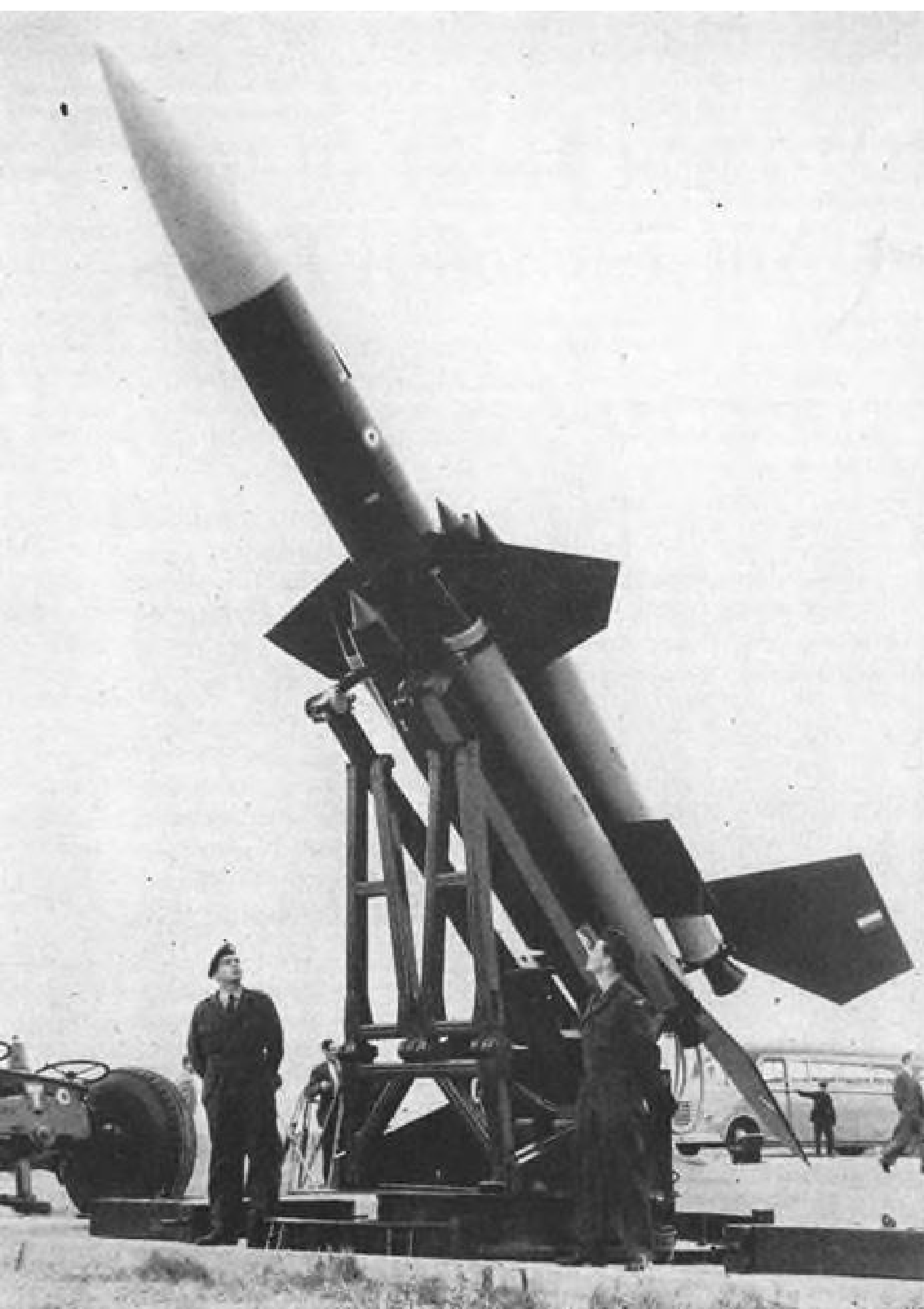
Positioning of Bloodhound's four booster rockets, two ramjets is shown (top right). Weapon stresses simplicity.
