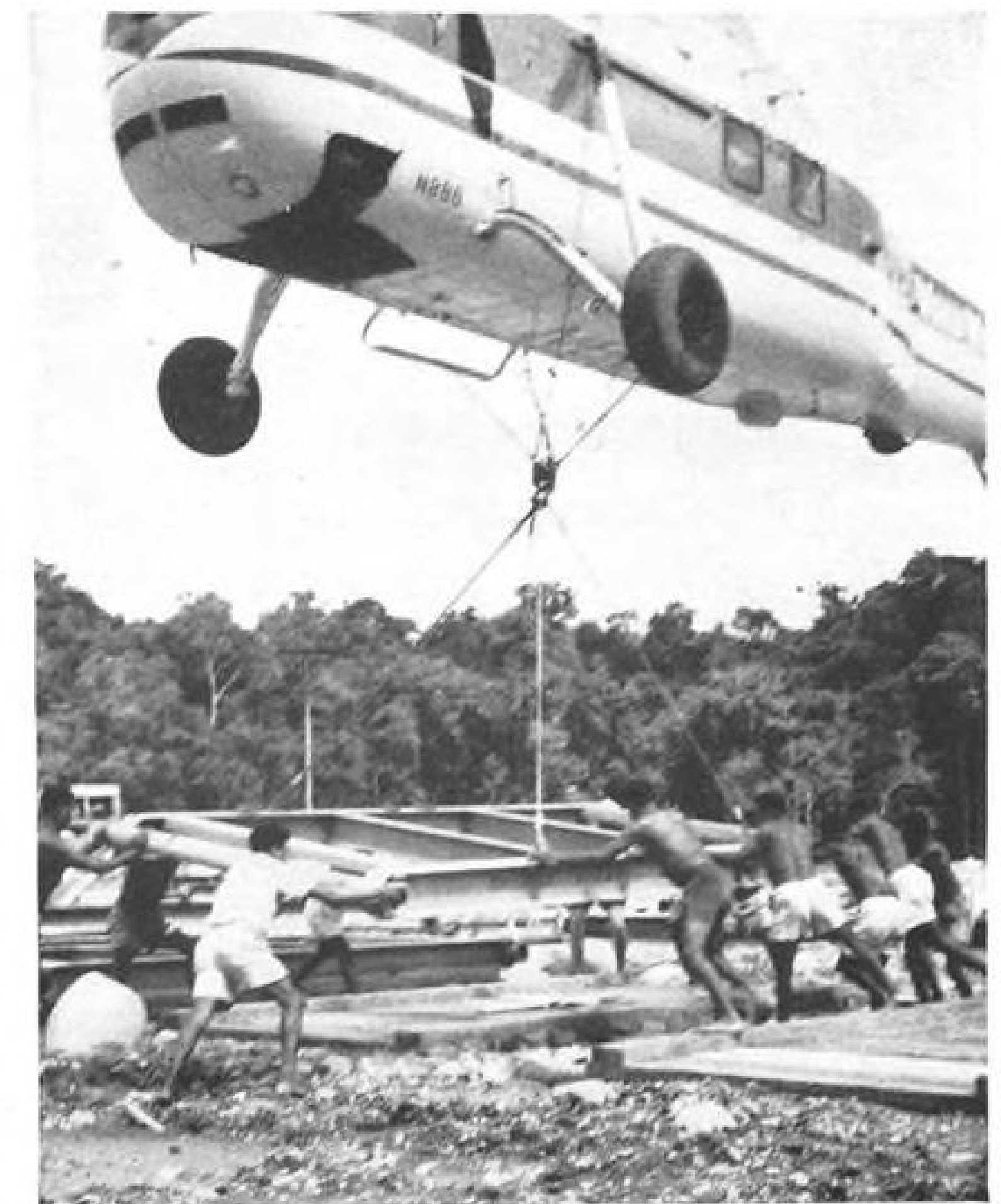
LEAVING river camp (left), S-58 starts for drilling site to deliver a load of lumber. Skid for drilling rig engines is swung into correct position for mounting by ground personnel (right). Helicopters can place some equipment in proper place for assembly.
