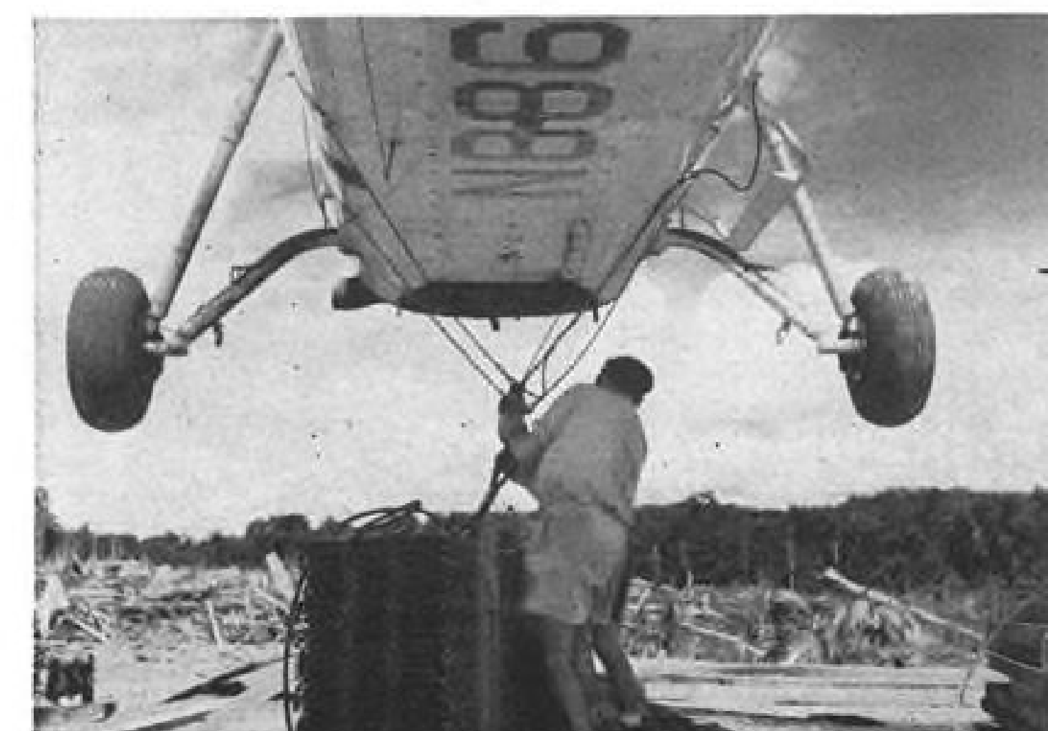
PIECED steel matting is hooked onto hovering S-58 (left). Ground crew (right) assembles S-58 at Port Moresby after sea trip from U.S. Helicopters were sprayed with plastic for protection at sea and first two S-58s delivered went through typhoon without damage.
