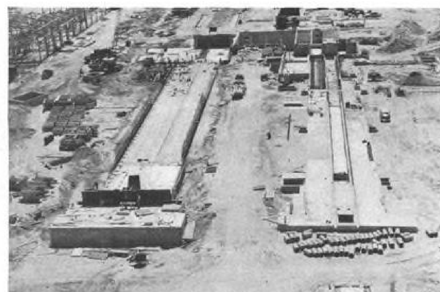
POWERHOUSE framework is shown (left). Aerial photo (right) shows C13 steam catapult (left) and C14 air/gas catapult construction progress. Note how C13 installation is raised 6 ft. above runway.
