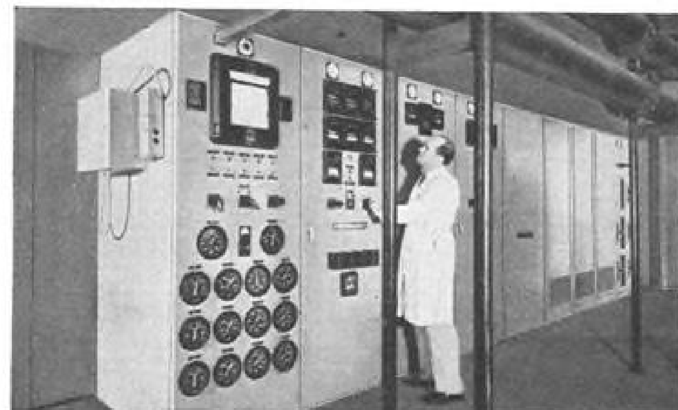
Allis-Chalmers also supplied switchgear and control for power distribution and protection.
