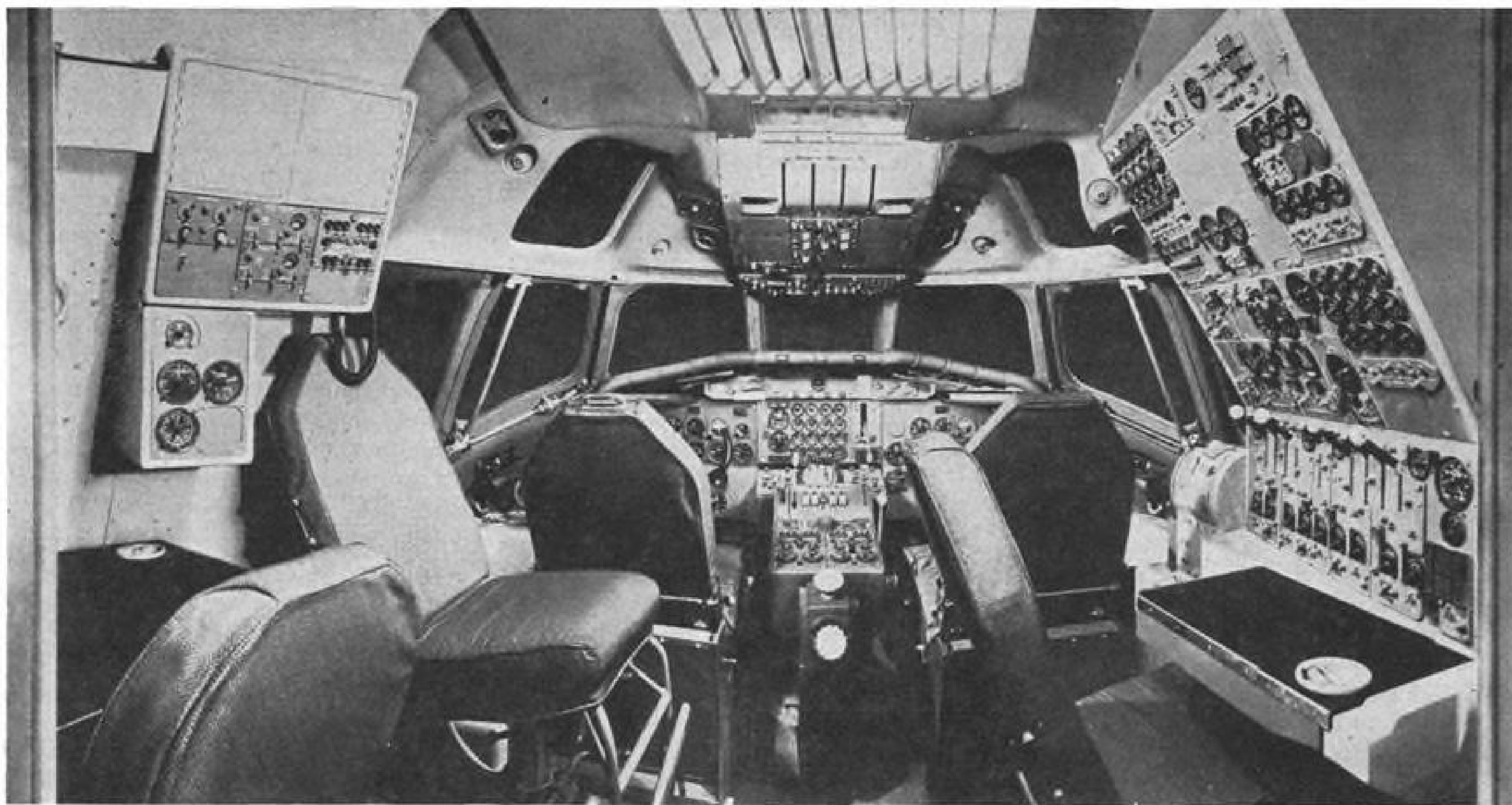
DC-8 COCKPIT mockup shot with flight engineer's station at right was union exhibit at emergency hearing.
