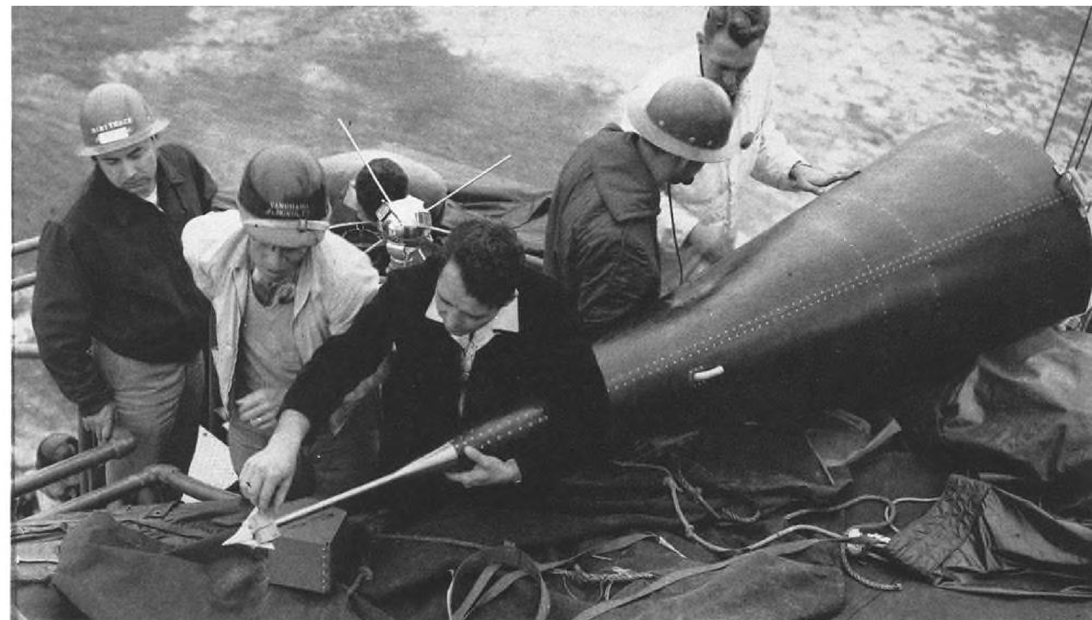
PROBE which measures Vanguard rocket angle of attack is adjusted by project engineers. Arrow-like device is attached to tip of asbestos phenolic plastic nose cone. Note actual 3.25 lb. satellite sphere undergoing checks at left center of picture.
