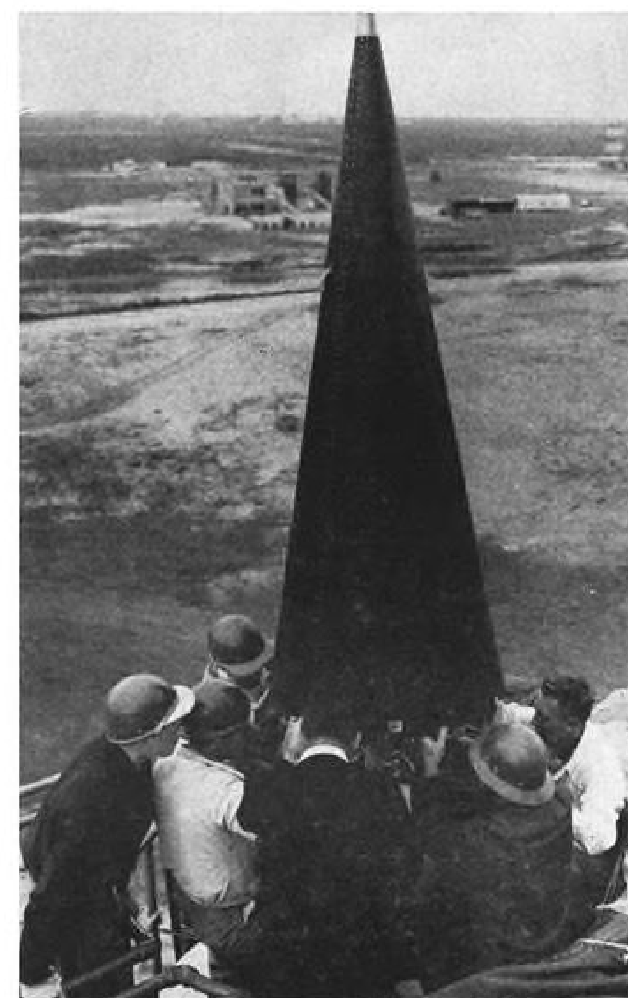
Vanguard nose cone is lowered into position (left), and inspected (center) by technicians. Nose cone is made of plastic phenolic; it streamlines vehicle and insulates sphere from heat. At right the gantry crane moves back and the satellite vehicle is cleared for firing.
