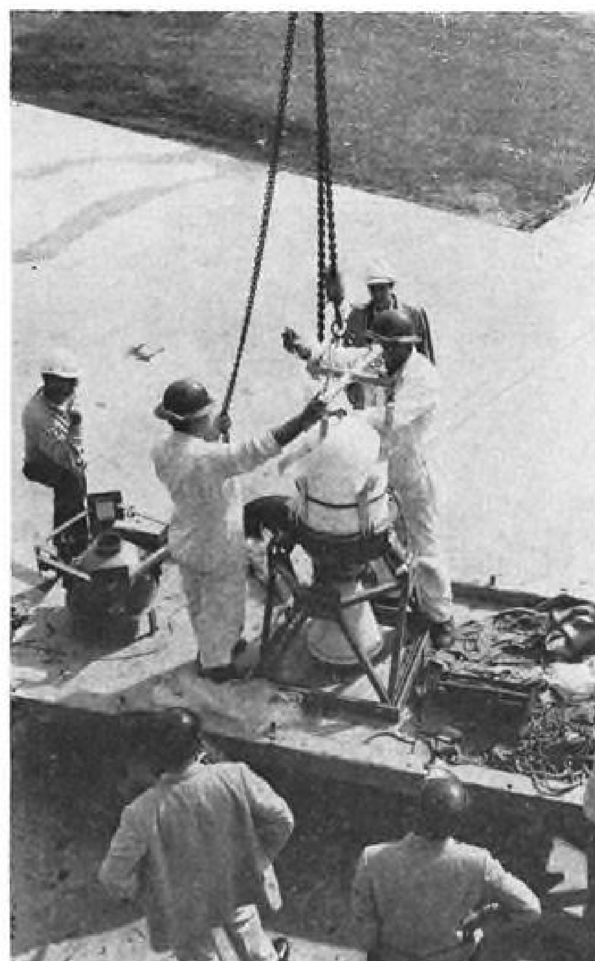
Third stage rocket of TV-4 Vanguard vehicle arrives at Cape Canaveral launching pad (left). Plastic film protects rocket from humidity. In center, propulsion unit is stripped of its protective packaging and is readied for hoisting. Vanguard is shown at right in shield.
