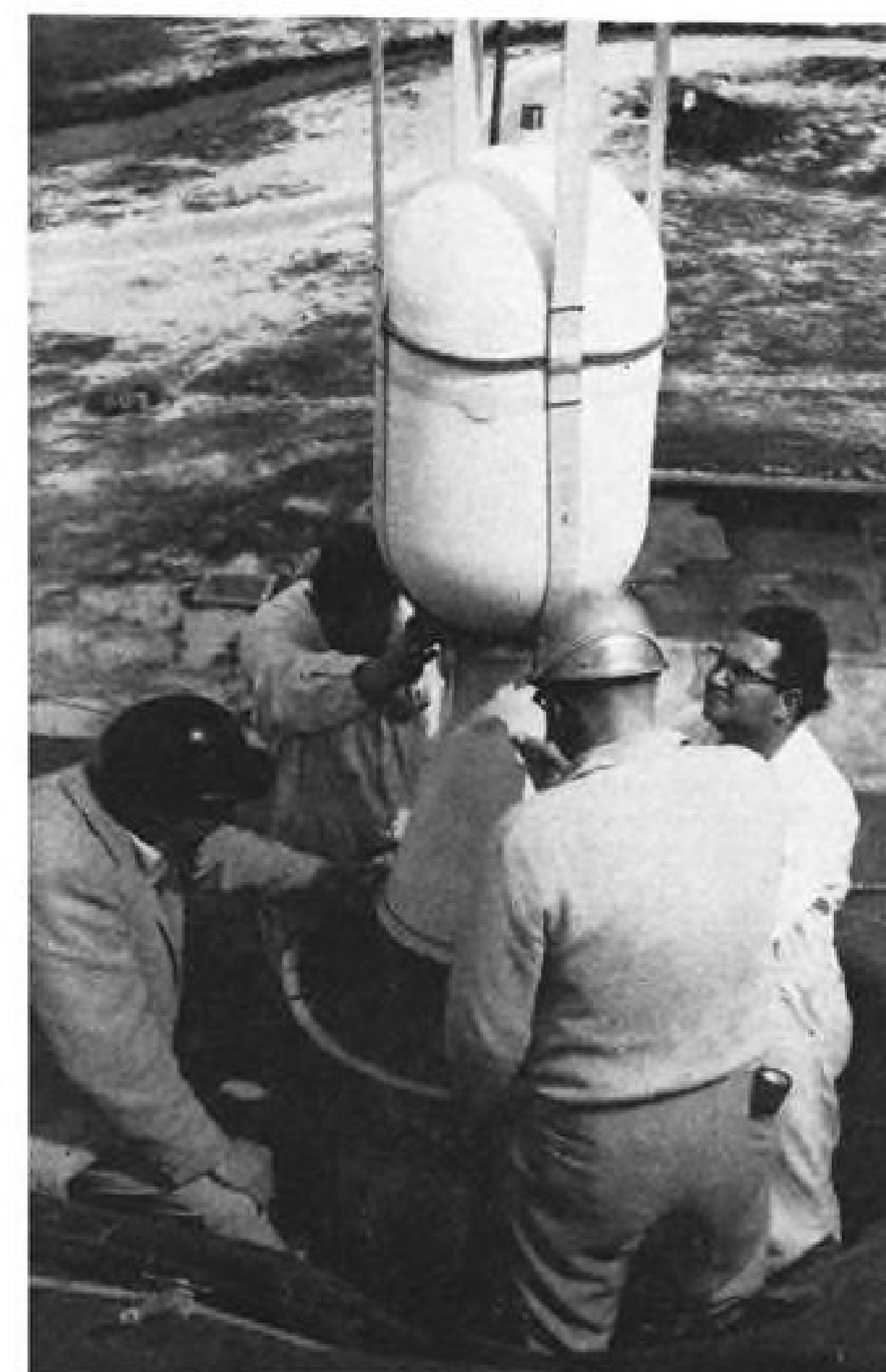
Third stage rocket is lowered into place, supported by sling (left and center). At right, engineers install spider guide on top of the third stage rocket. Spider guide is designed to steady the rocket unit so that separation from vehicle is straight and accurate.
