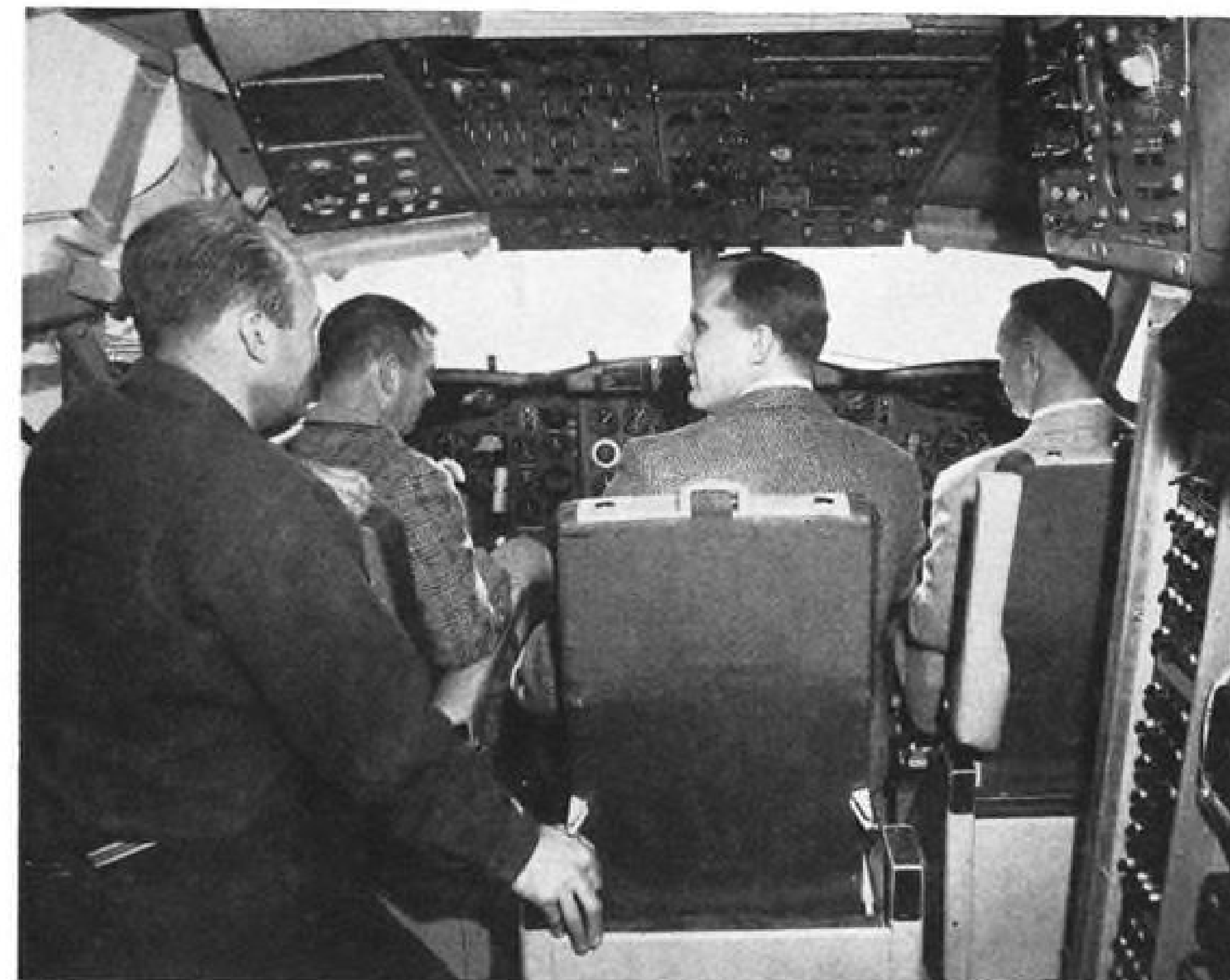
VISIBILITY is good in Electra cockpit, which has three-abreast seating. Flight station has separate air conditioning system, also has 11 cu. ft. portable oxygen cylinder for crew use.
