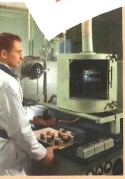
SPECTOGRAPH analyzes materials both quantitatively and qualitatively to an accuracy of one part in one-million! The spectrum of a blinding arc of the material is recorded photographically for analysis.
