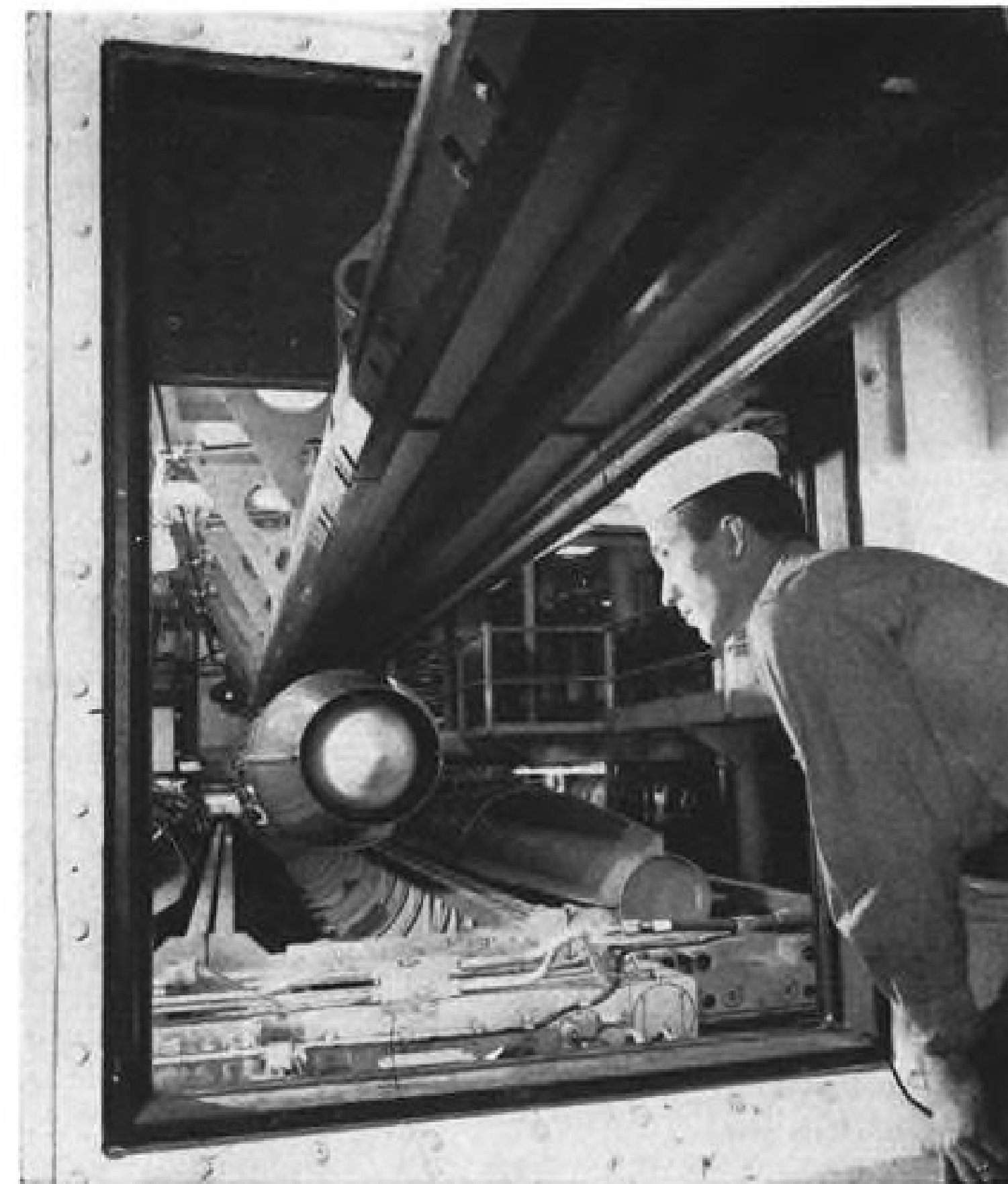
SUPERSONIC Bendix-Talos ramjet-powered guided missile is carried aboard U. S. Navy cruiser Galveston (left), which was commissioned last week at Philadelphia. Missile, built by Bendix Aviation Corp., has range of more than 65 mi. At right, missile in foreground is nuclear armed with "clean" nose except for pitot line visible in photo. Talos in background is conventional version which uses semi-active guidance for homing on target, has four antennas located 90 deg. apart around periphery of nose. Several other ships will be fitted with Talos.
