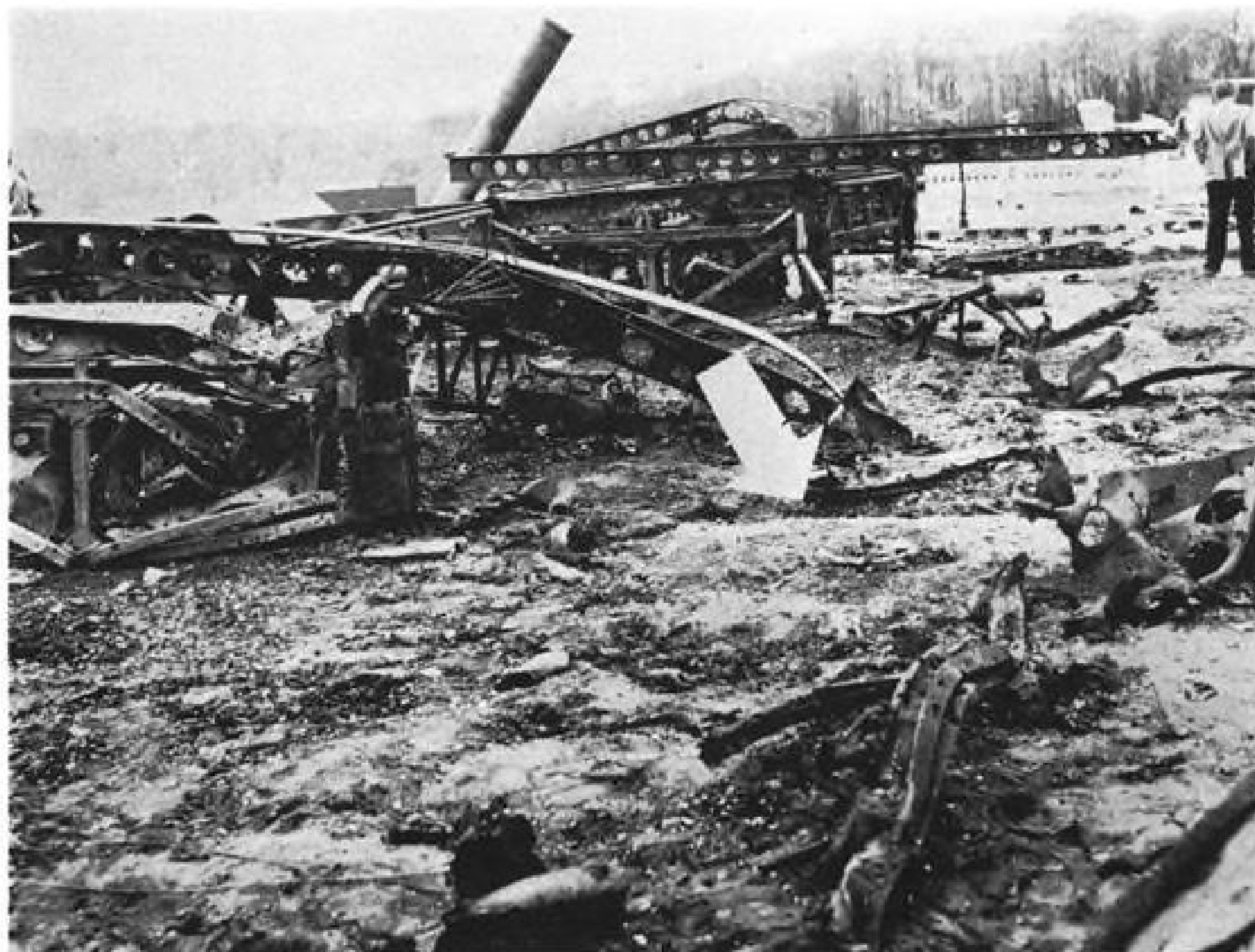
ALPHA SECTION seen from direction of the Assembly building. Explosion apparently originated between launching position four at far left and launching position three at center. Arrow points to crater about three feet deep where nose and center warheads removed from missile that was being modified are believed to have been placed. Metal framework has all been extensively perforated by pellets from exploding warheads.
