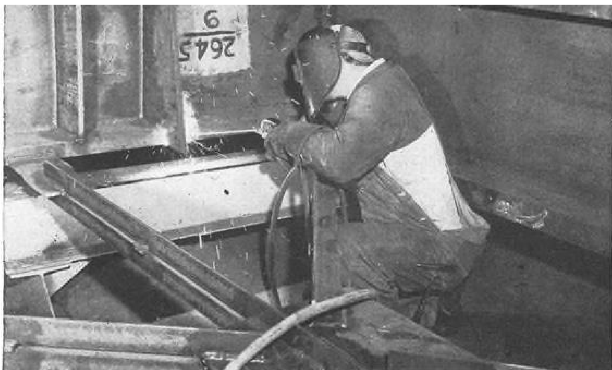
Erector towers for USAF's Titan intercontinental ballistic missile are being constructed at Kaiser Steel Corp.'s Steel Fabricating Plant at Montebello, Calif. Above, heavy steel section of basic tower structure is welded. The Martin Co. is prime contractor for Titan.
