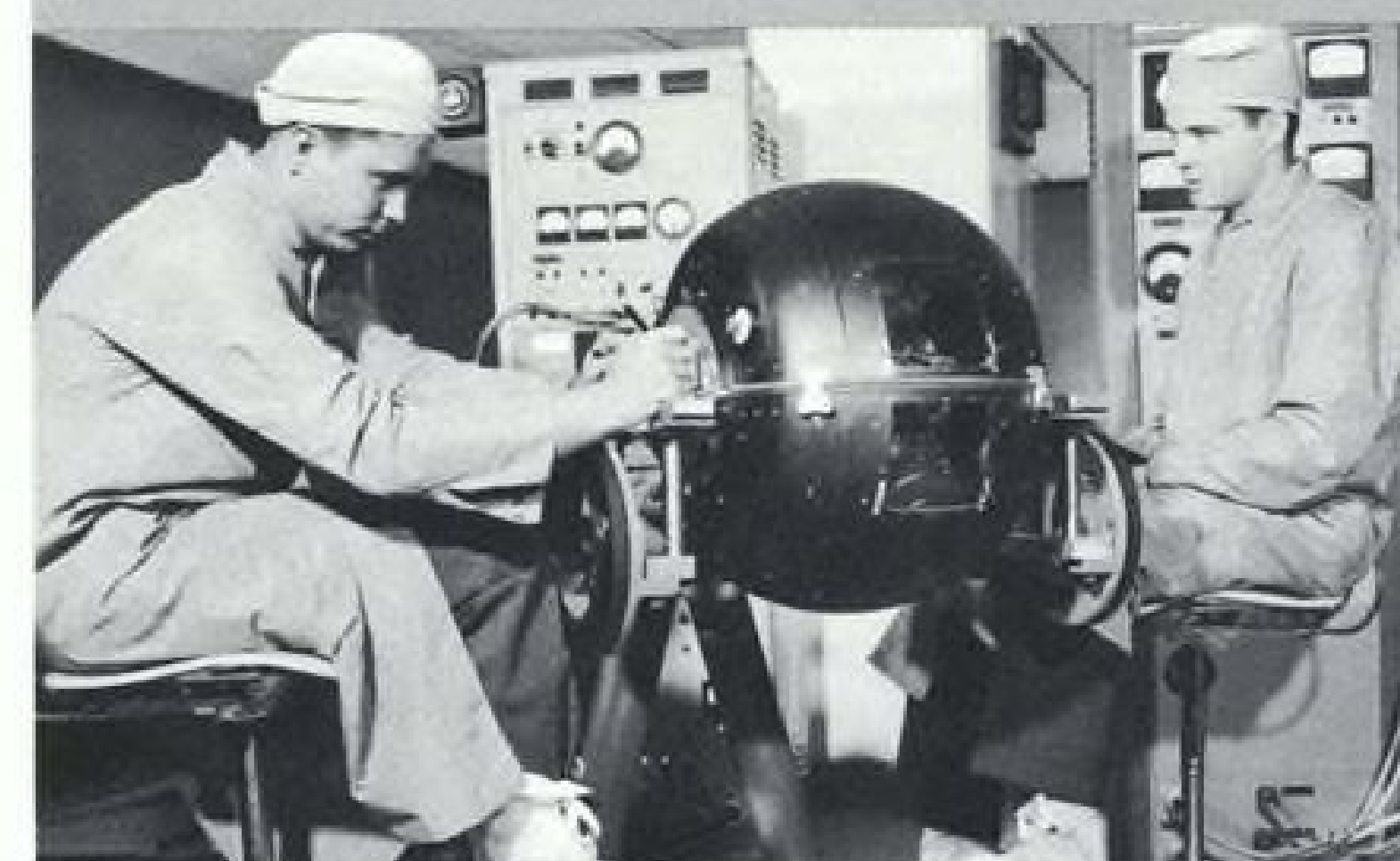
Stable platforms. Technicians here are performing test operations on a stable platform for the U. S. Army JUPITER Missile; these platforms are in quantity production at Ford Instrument.
