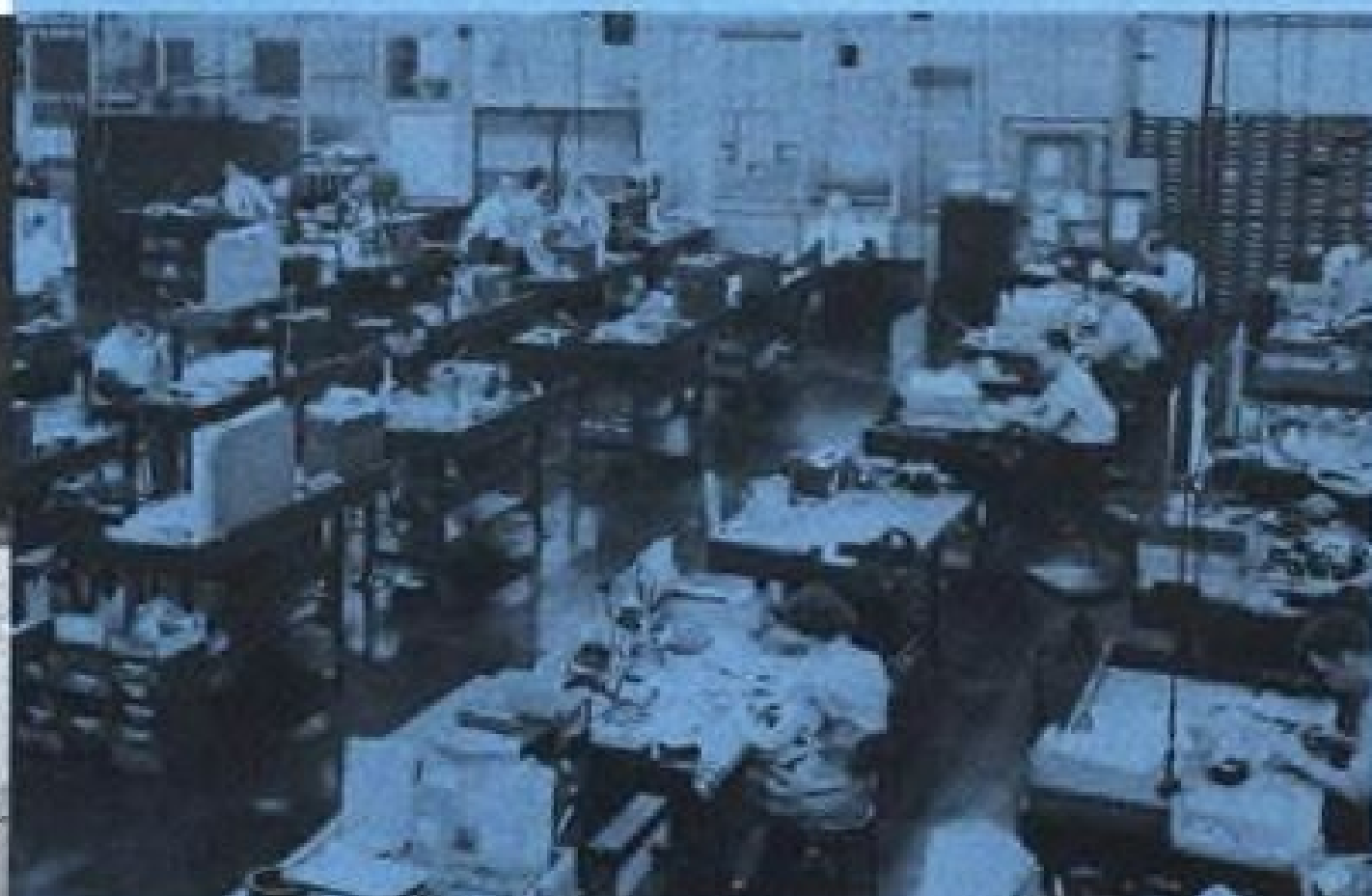
Engineering Shop. This shop makes breadboard models and other experimental products. It has much specialized equipment, e.g., toroidal coil winders, lapping equipment, in addition to standard machine tools.
