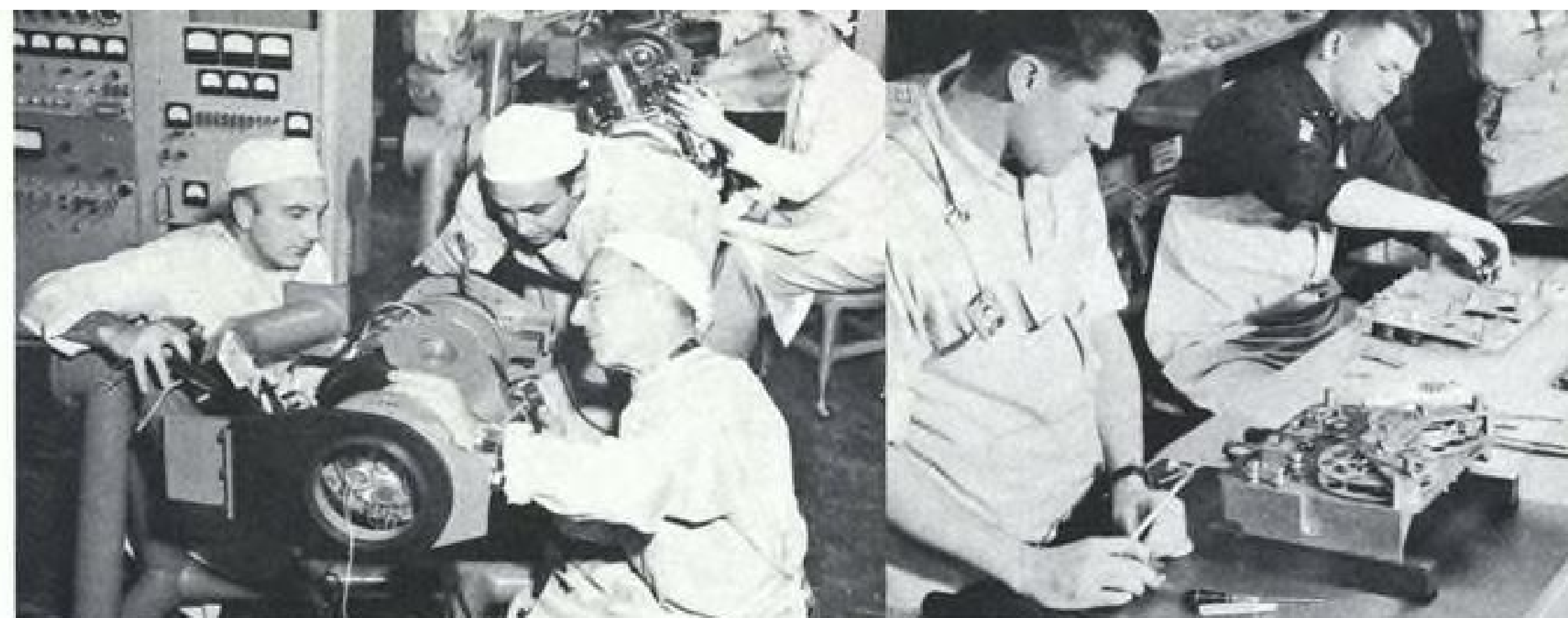
Missile-borne tape programmers being assembled. Continuous development in this field is under way at Ford.
