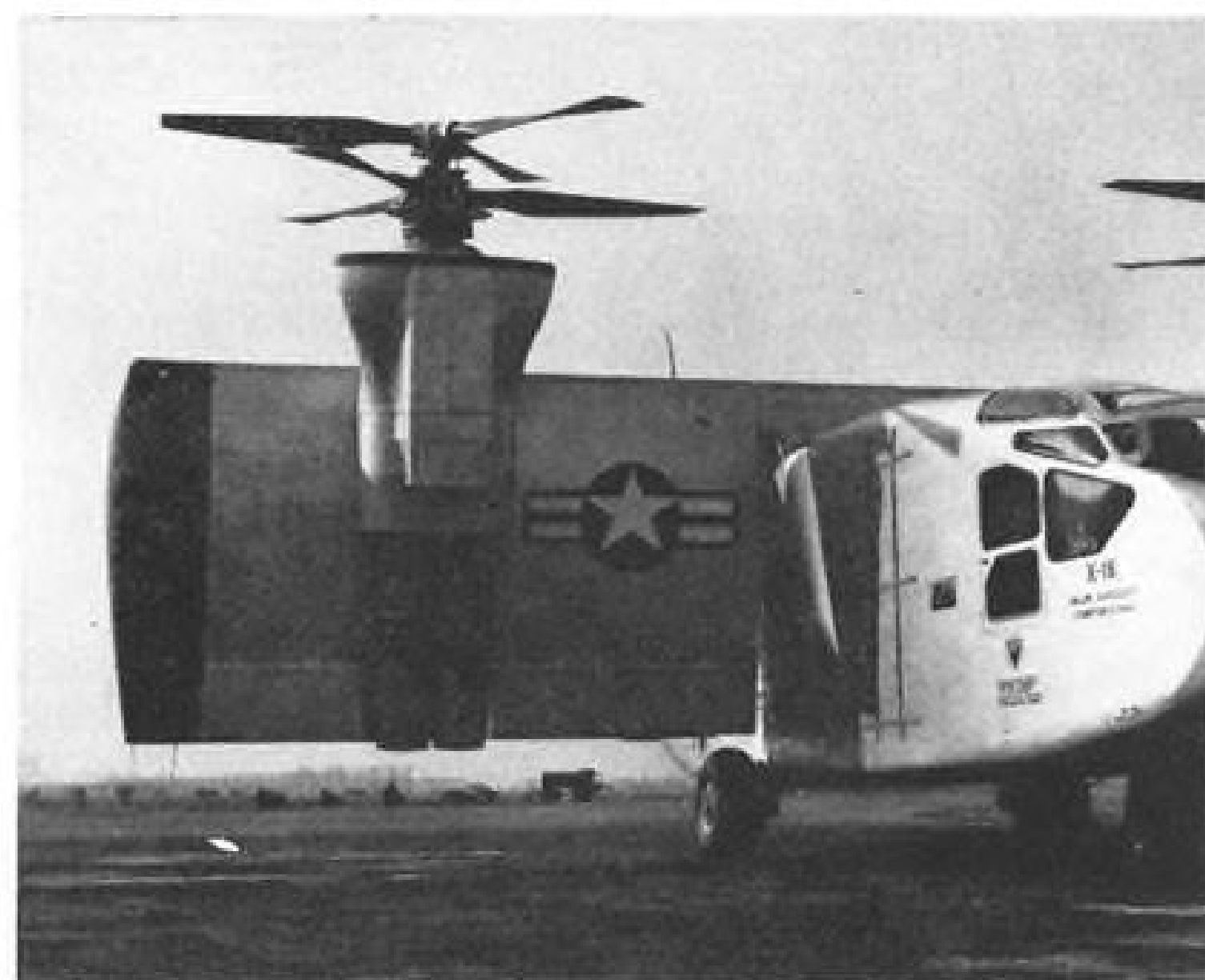
NOSE AND TAIL sections are adapted from Fairchild C-123 transport; note horizontal stabilizer dihedral. Propellers are dual-rotating Curtiss-Wright turboelectric unit from Navy Pogo VTOL program.
