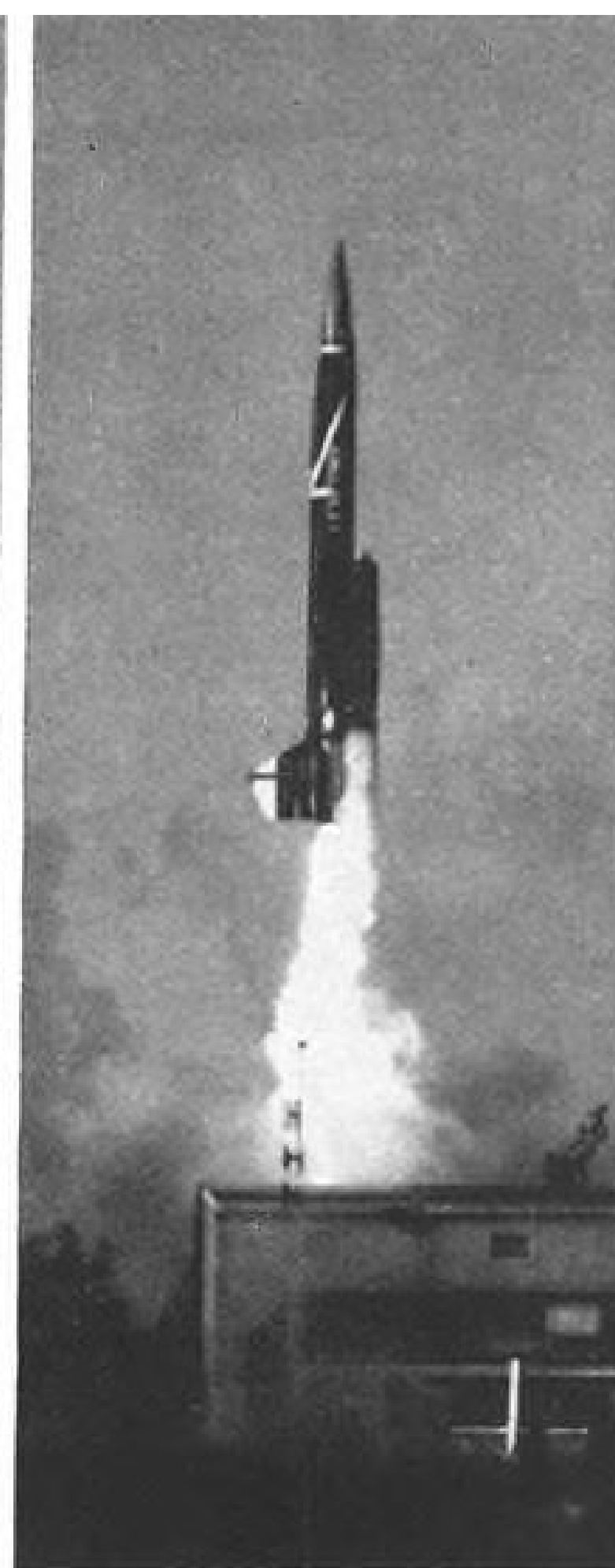
BOMARC IM-99A climbs vertically from launching enclosure after firing, stabilized in this phase by its gimbaled booster engine
