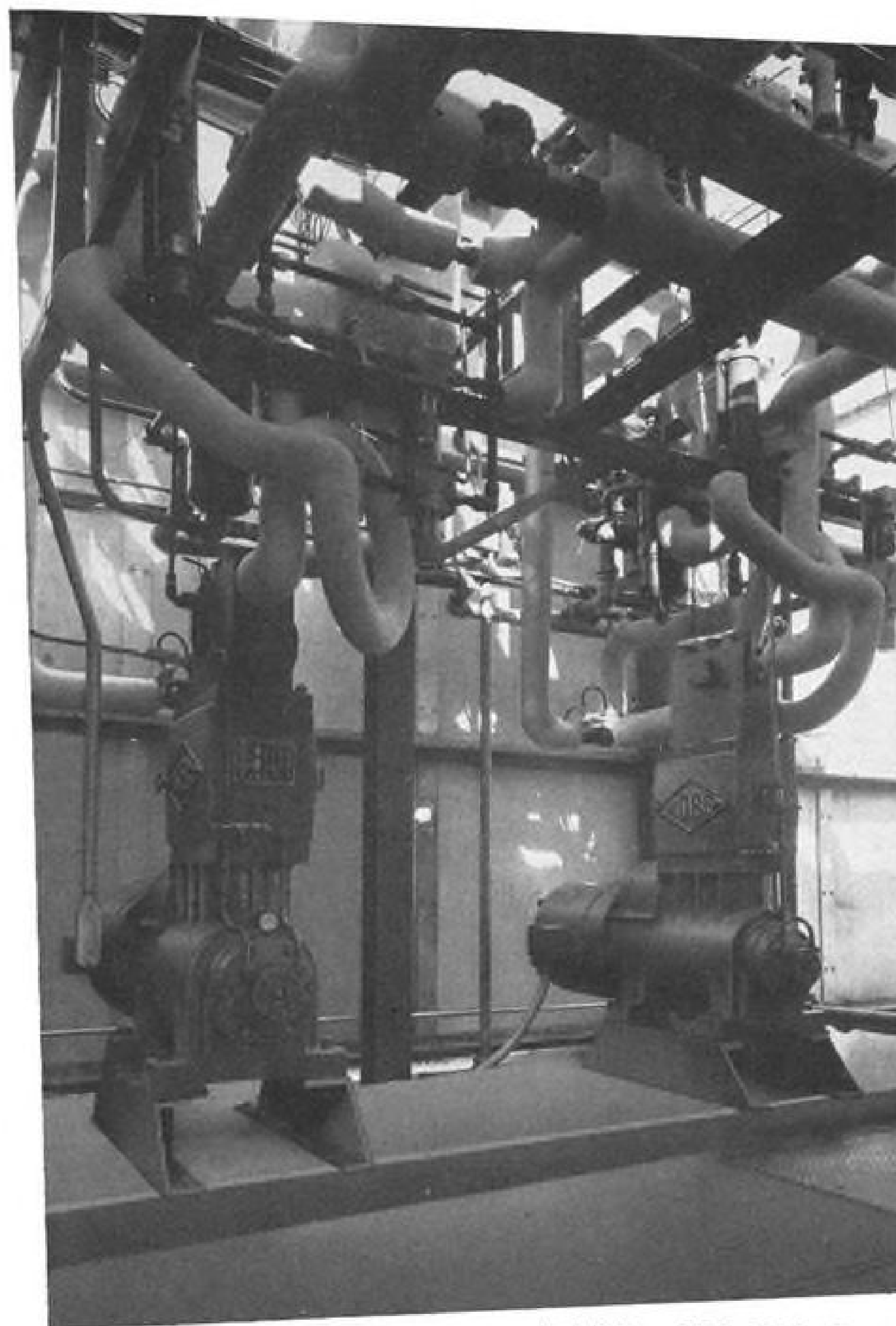
Installation of Kobe Triplex Pumps at the Bendix-Pacific high temperature facility
