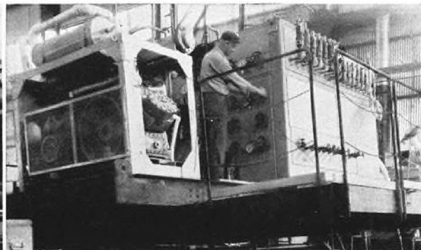
Shipboard liquid oxygen—liquid nitrogen generator. Air Products successful development of units like this was a major technological breakthrough in cryogenic equipment design. More than 40 are now aboard U.S. Navy vessels. This one . . . rated at 1.3 tons per day of high purity oxygen . . . is being tested on a special rig that duplicates the rolling and pitching motion of a ship.
