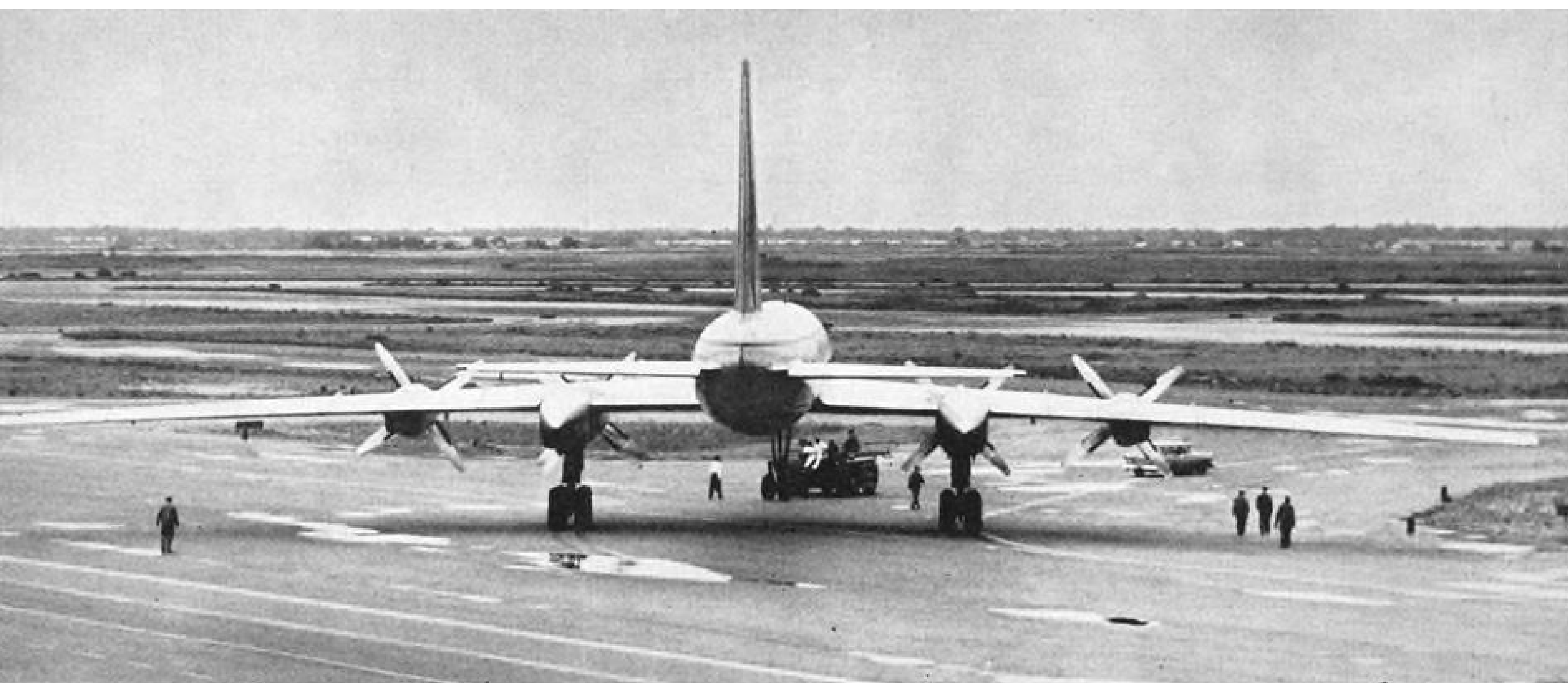
BEING TOWED to taxiway at N. Y. International Airport for engine runup, Tupolev Tu-114 shows clean cross-section in rear view, marked negative dihedral of its swept wings. Huge size is apparent when compared with personnel walking turboprop transport to taxiway.
