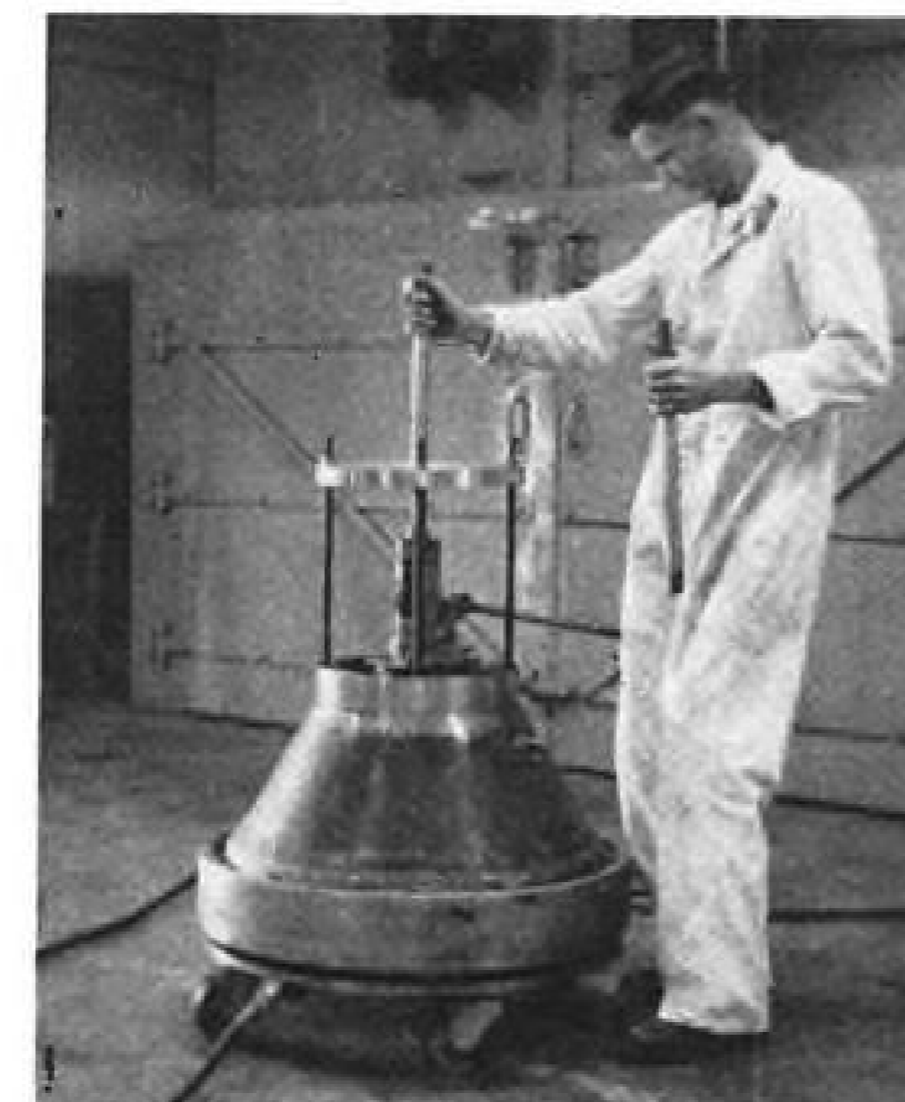
Aft head is placed in assembly to vulcanize rubber-based insulation to inside (left). At center, the rocket motor has been removed from casting bell for application of the nozzle assembly. Special jig (right) is used to align aft head assembly to rocket case.
