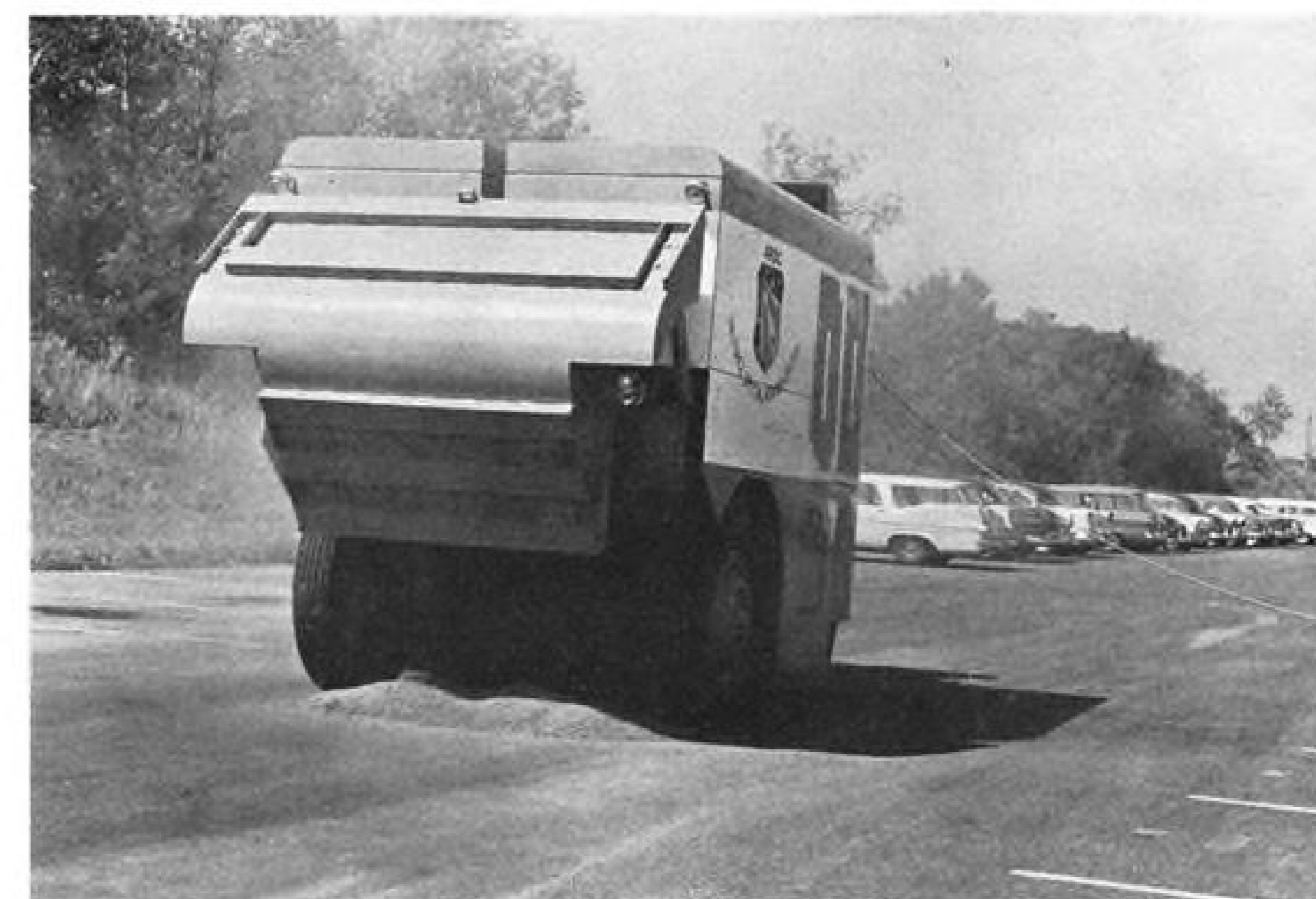
SWEeper demonstrates its time-cycled automatic dumping operation. The 4 cu. yd. hopper is lifted to full height three times to dislodge all residue.
