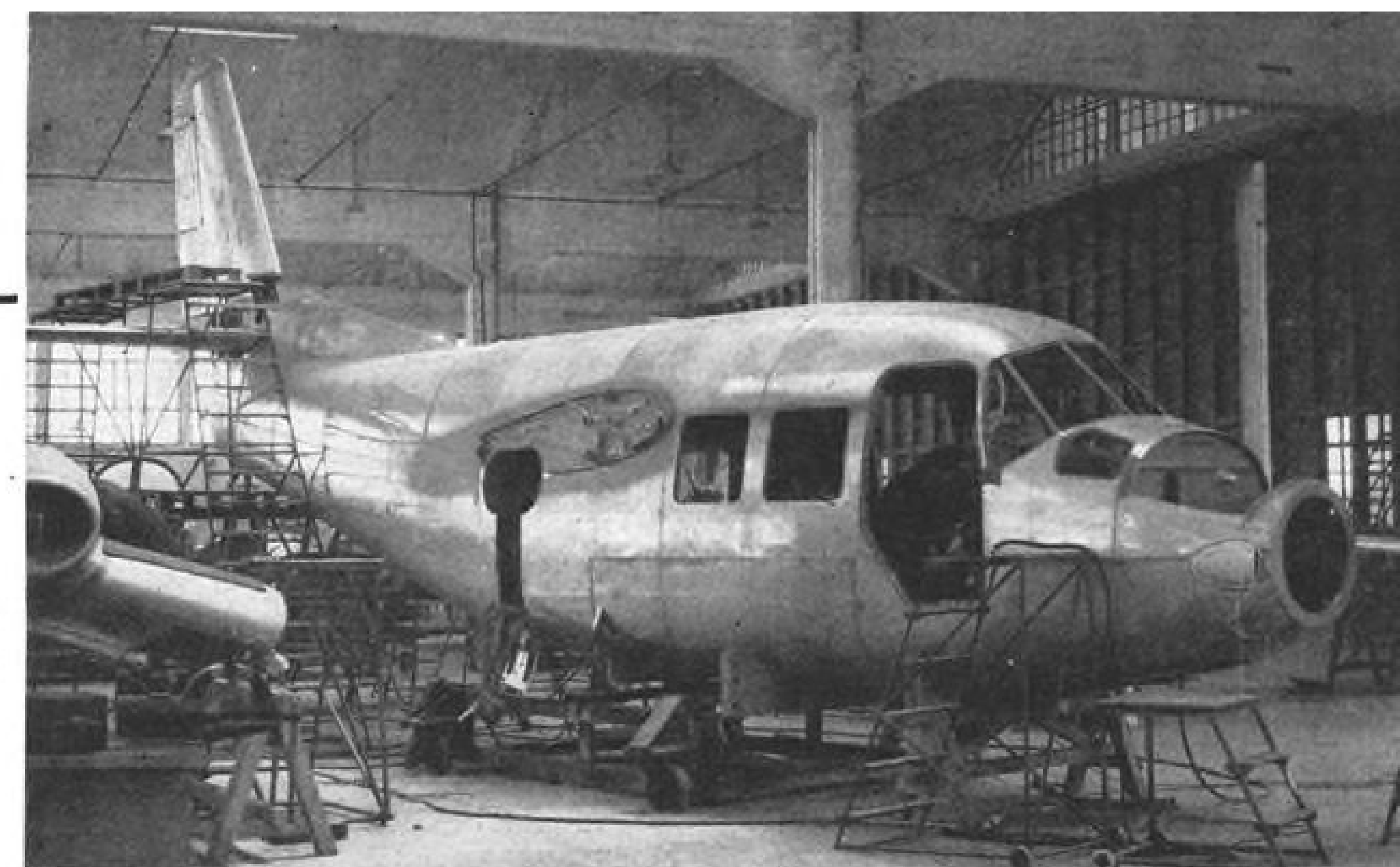
EXTERIOR VIEW of the P.166 fuselage points up aircraft's similarity to the amphibious P.136, from which it was derived. Structure is semi-monocoque, without longerons. Aluminum coated, flush-riveted light alloy skin is used throughout.
