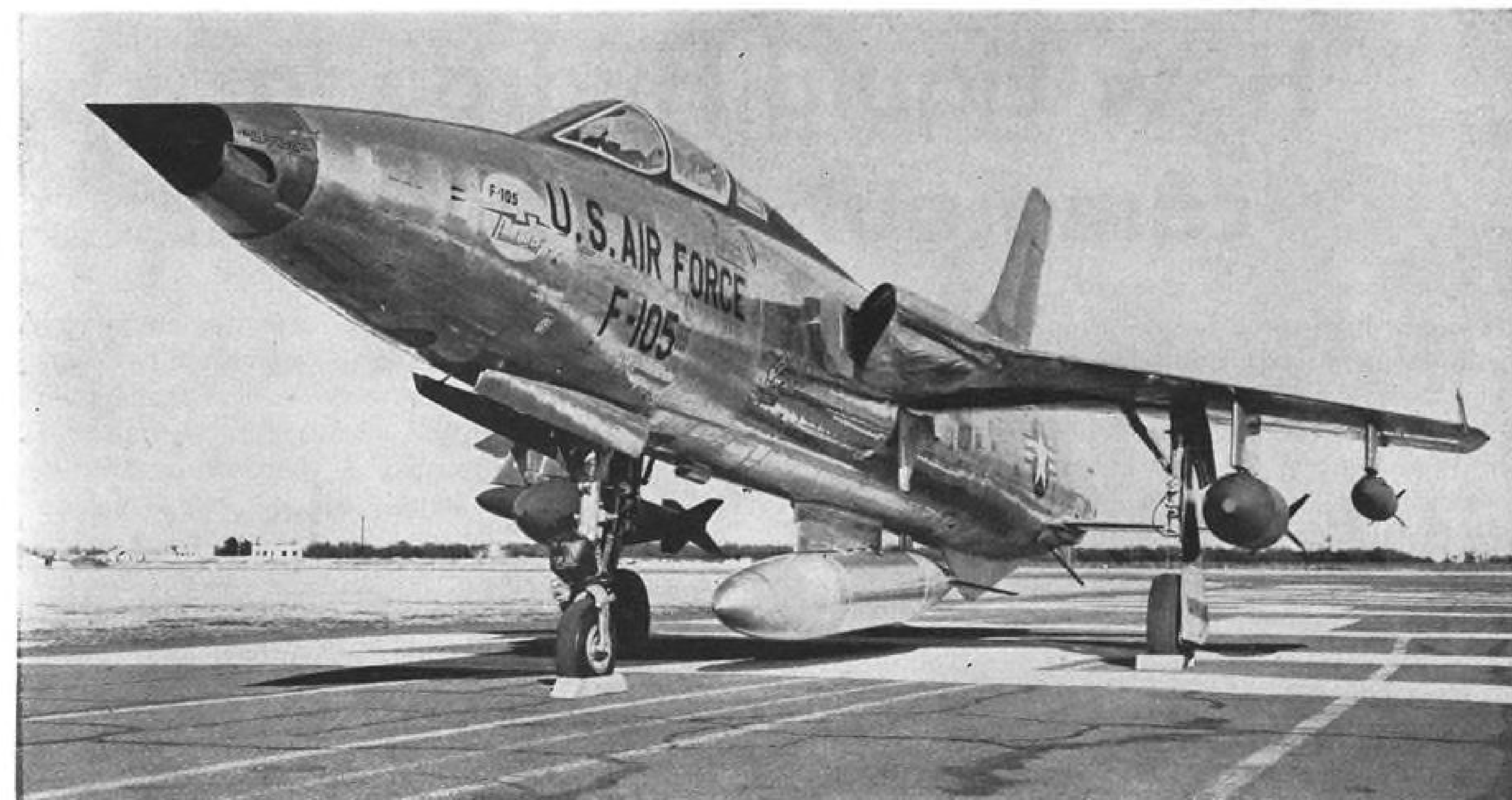
ARMAMENT carried by this F-105B at Seymour Johnson AFB includes two 3,000-lb. T-55 bombs outboard and two 750-lb. Mk.83 bombs inboard. Carried under the belly is a 450-gal. external fuel tank. Long bomb bay will carry a nuclear weapon.
