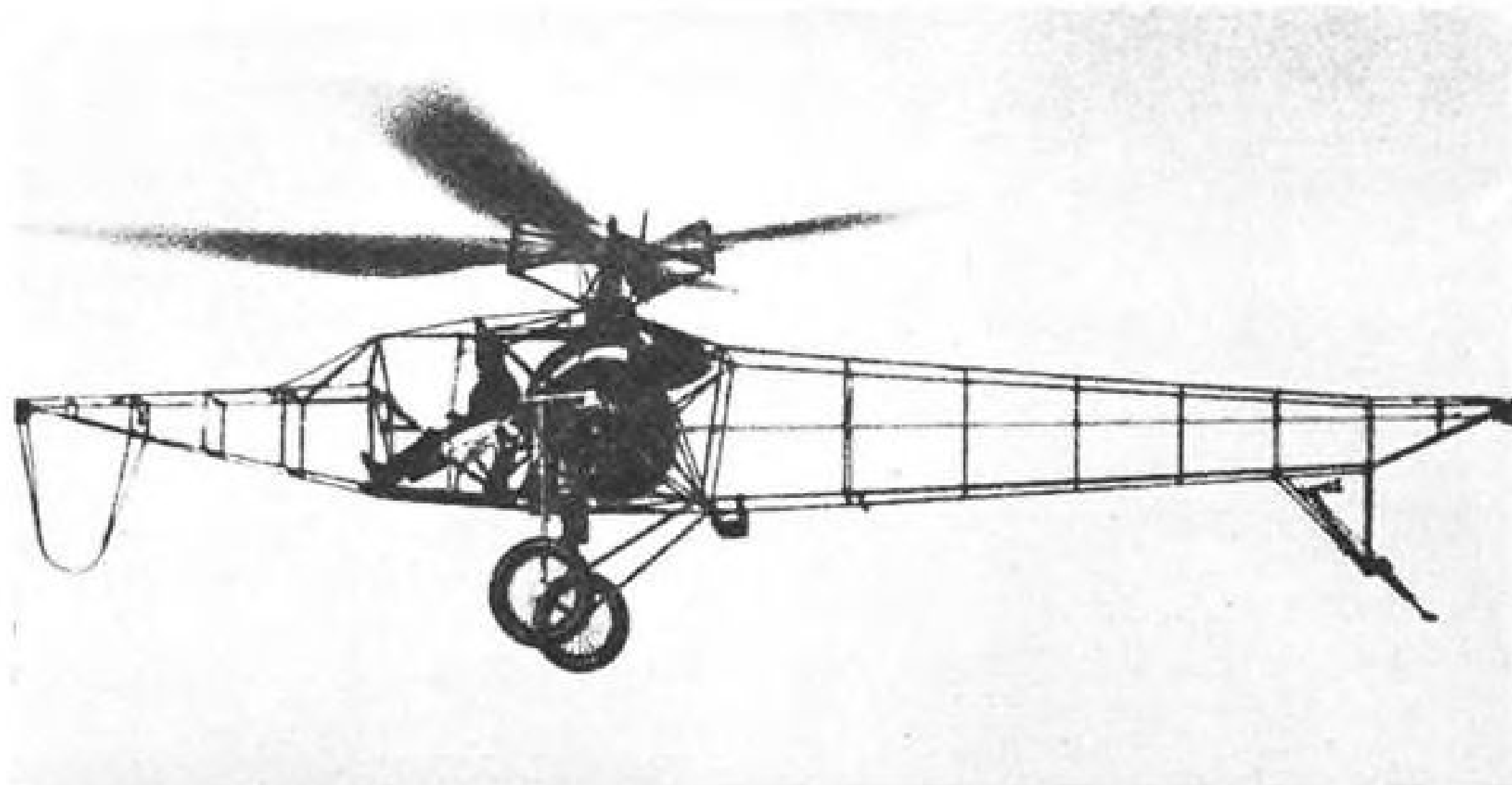
SINGLE-ROTOR helicopter developed in 1932 by the Zhukovsky Central Aero-Hydrodynamical Institute set a world altitude record of 605 meters (1,985 ft.). The Institute provided important assistance for the Yak-24 project.
