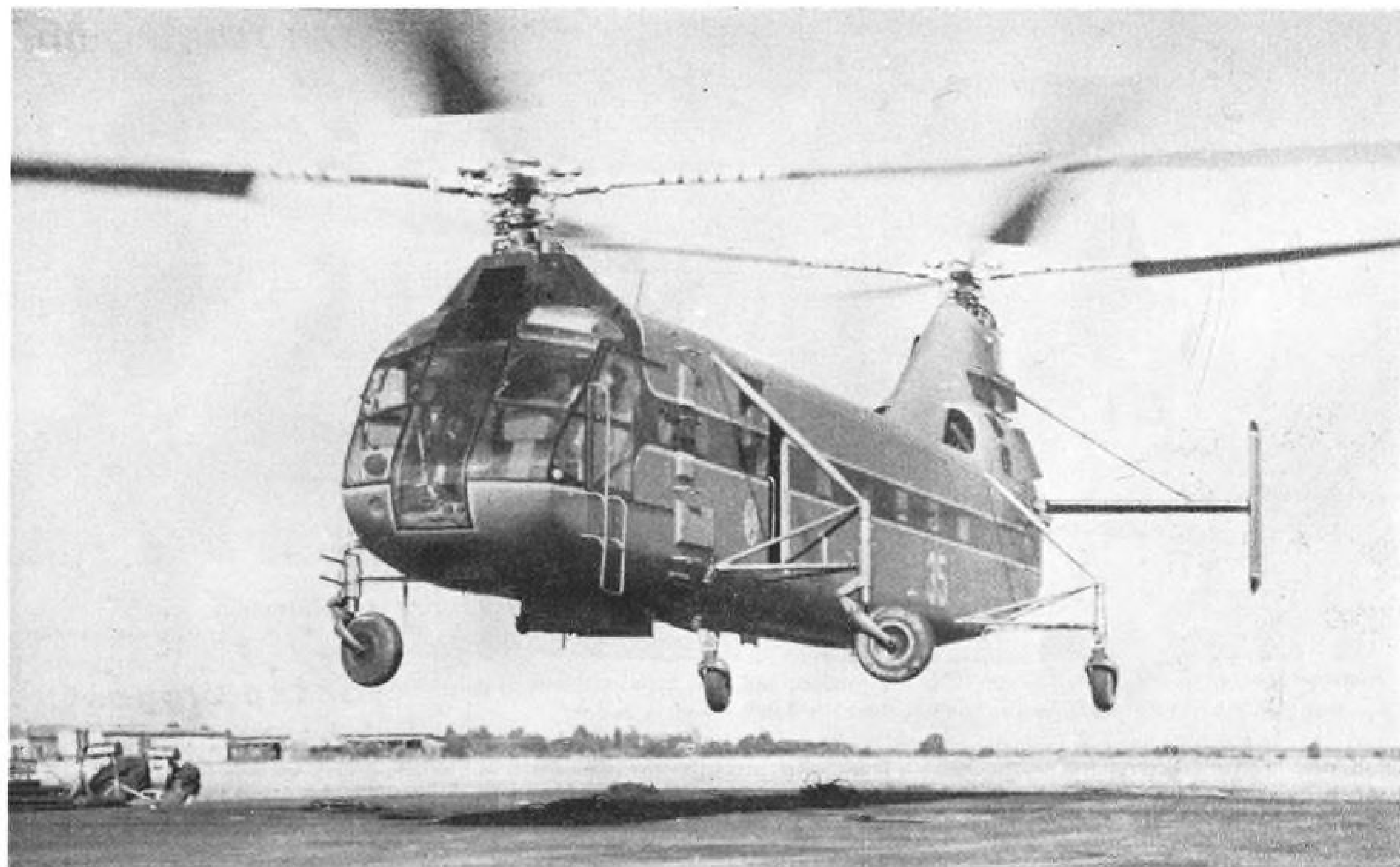
LONGITUDINAL arrangement for rotor positioning was used for the first time in the USSR on the Yak-24. The helicopter's navigational equipment permits it to make flights at night and under difficult weather conditions. The Yak-24 project was initiated in 1952.
