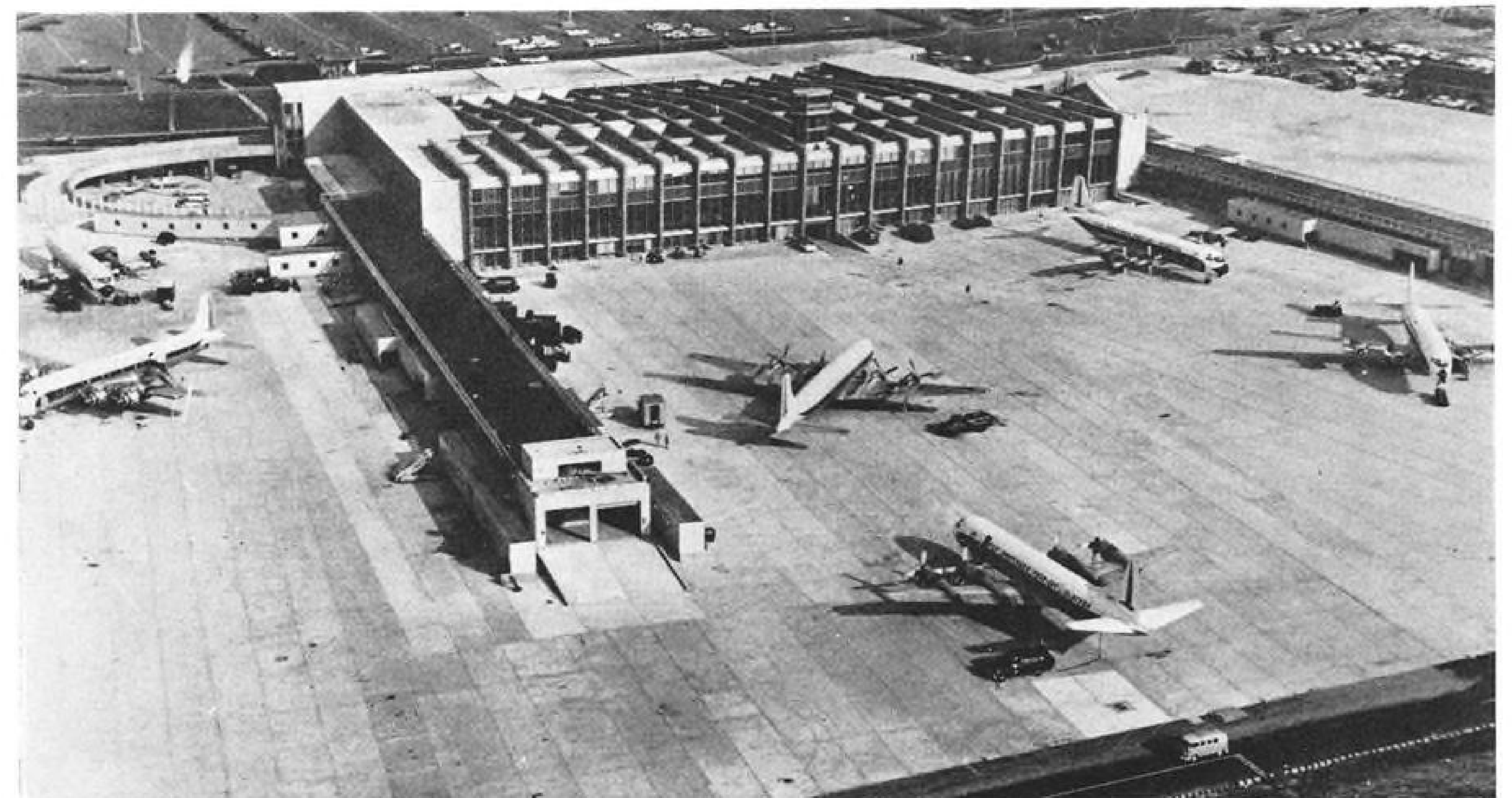
Eastern Air Lines' $20 million passenger terminal at New York International Airport has two 350-ft. passageways which provide 16 gates. Twenty-four aircraft can be parked simultaneously on the apron. Terminal is used by 104 daily inbound and outbound flights.
