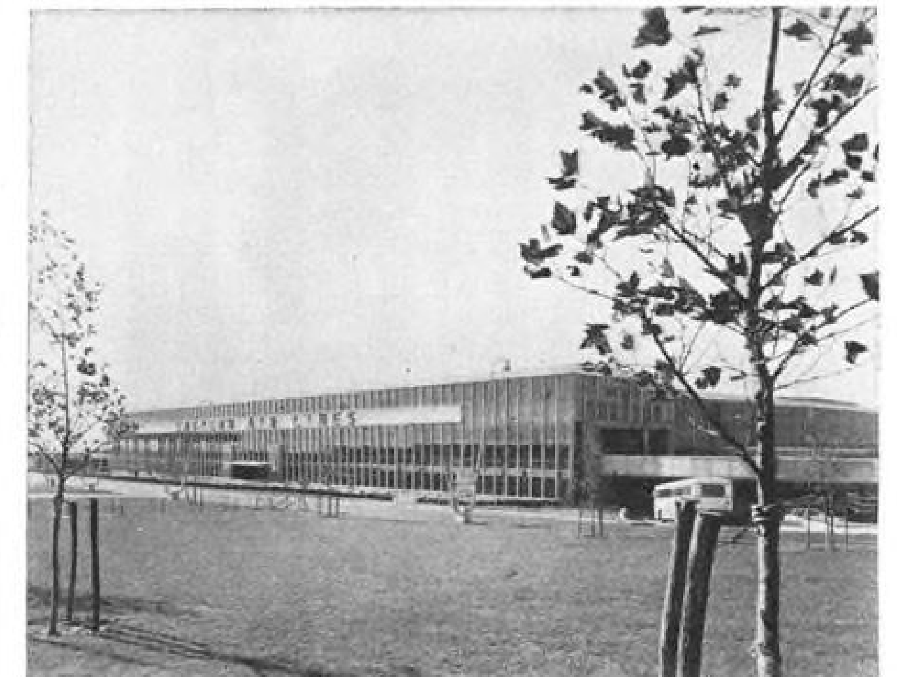
All major Idlewild runways and taxiways and all loading and unloading Eastern aircraft are visible from 83-ft. high coordinator's tower (above, left). Coordinator controls all movement of aircraft and ground vehicles on terminal's apron area, and controls passenger information. Upper and lower vehicular driveways are enclosed behind 375-ft. facade (above, right). Main lobby is on second floor (below, left); zig-zag pedestrian ramps (below, right) connecting first and second levels are hung from stainless steel cables.
