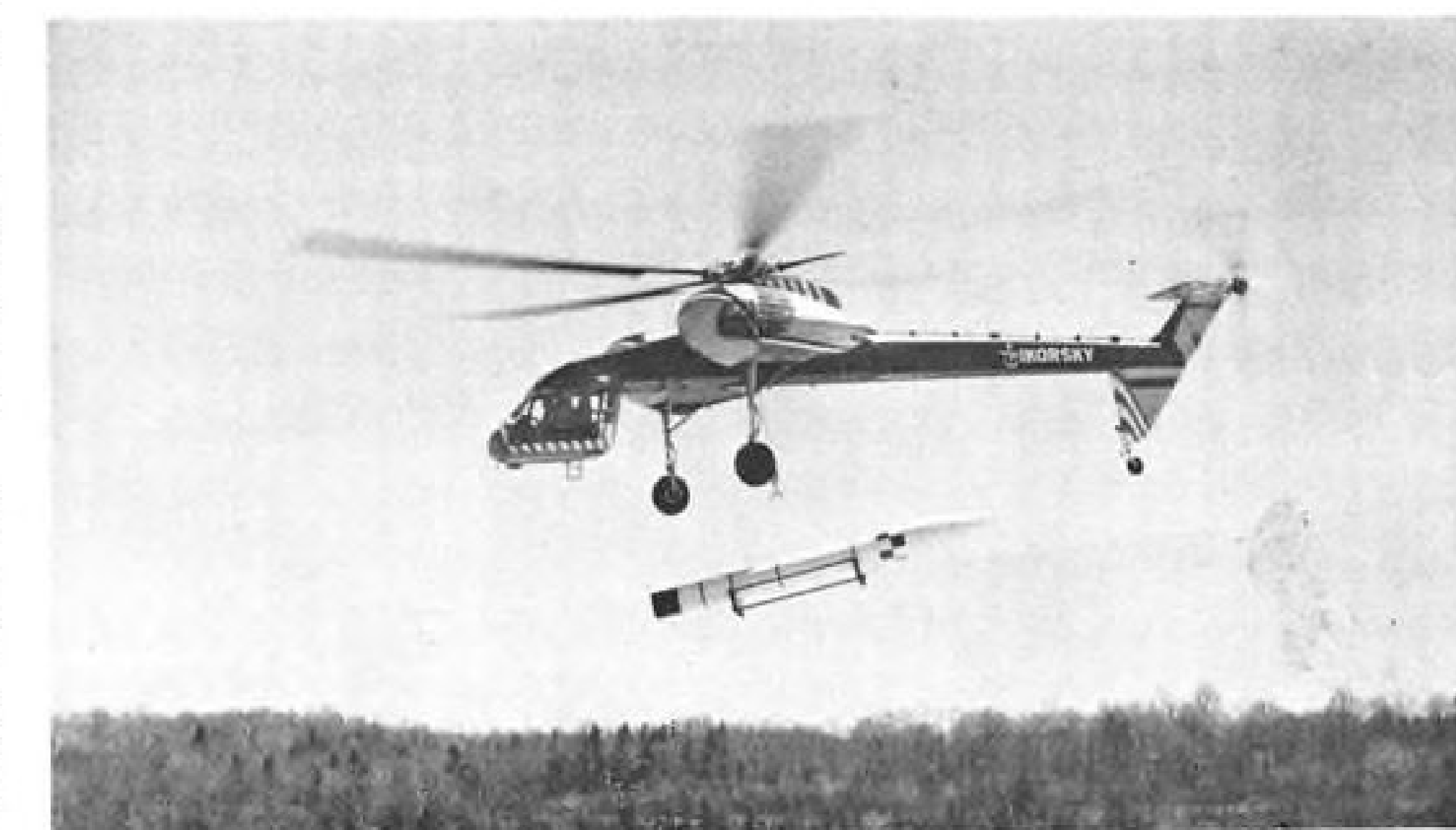
MOCKUP of Honest John rocket, with fins removed, is airlifted by S-60. The helicopter can haul a five-ton payload and cruise at 100 kt. Still-air range is 230 naut. mi.
