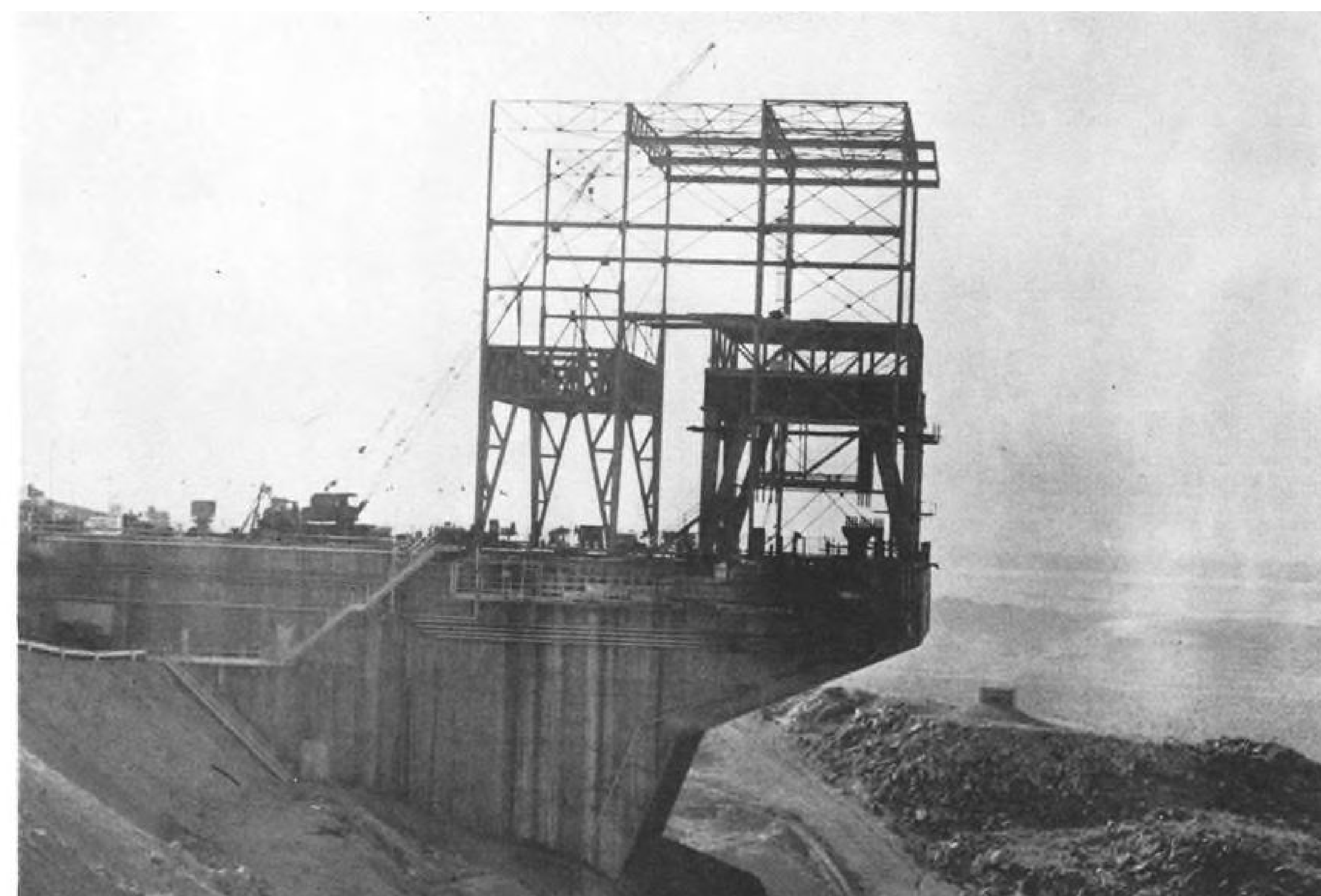
TEST STAND for NASA-Rocketdyne F-1 1.5-million-lb.-thrust engine was designed primarily by a division of Aerojet under Army contract.
