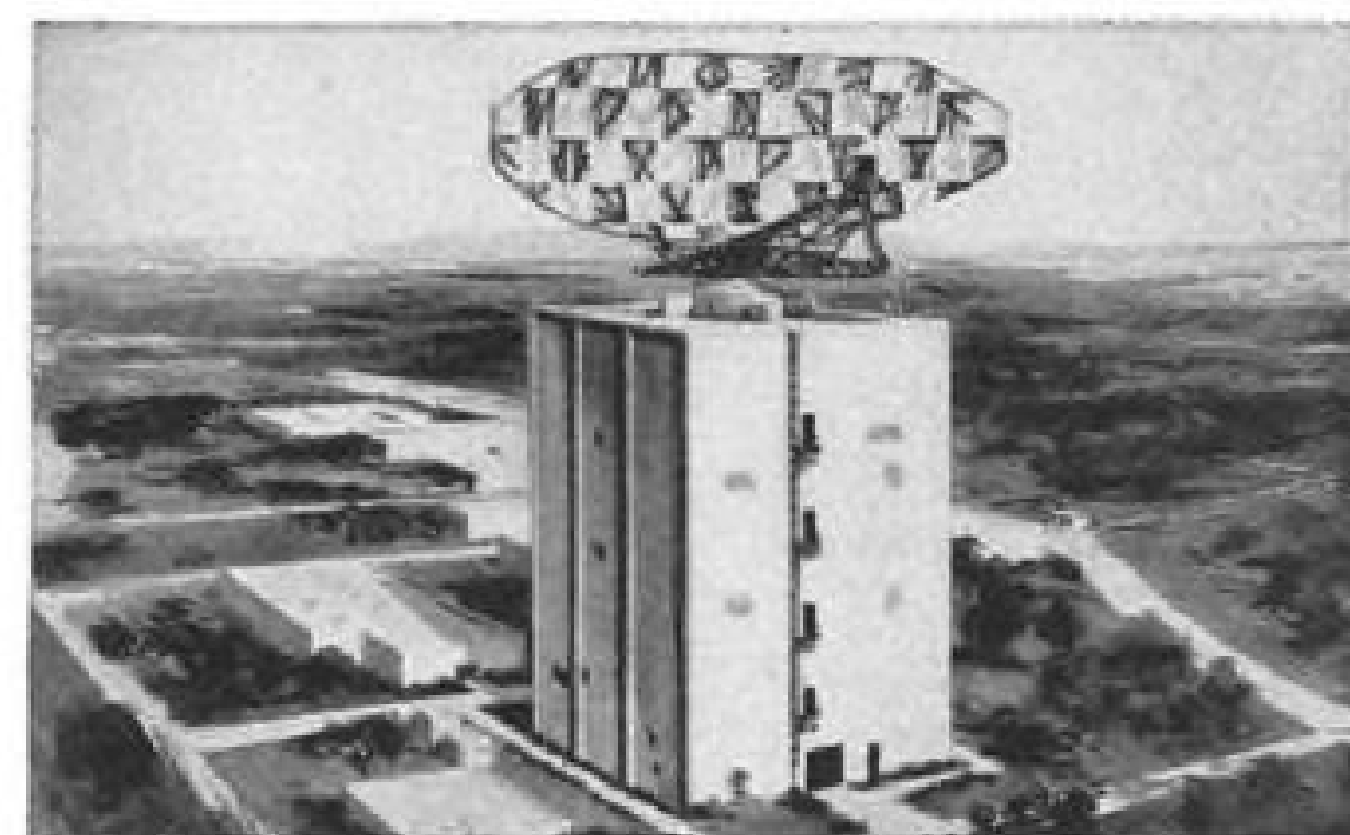
TOWER OF STRENGTH in U.S. defenses is strategic network of huge radars for warning of incoming missiles and aircraft. Developed by Sperry in cooperation with the Air Force, system has 70-ton antenna, 85-foot tower.
