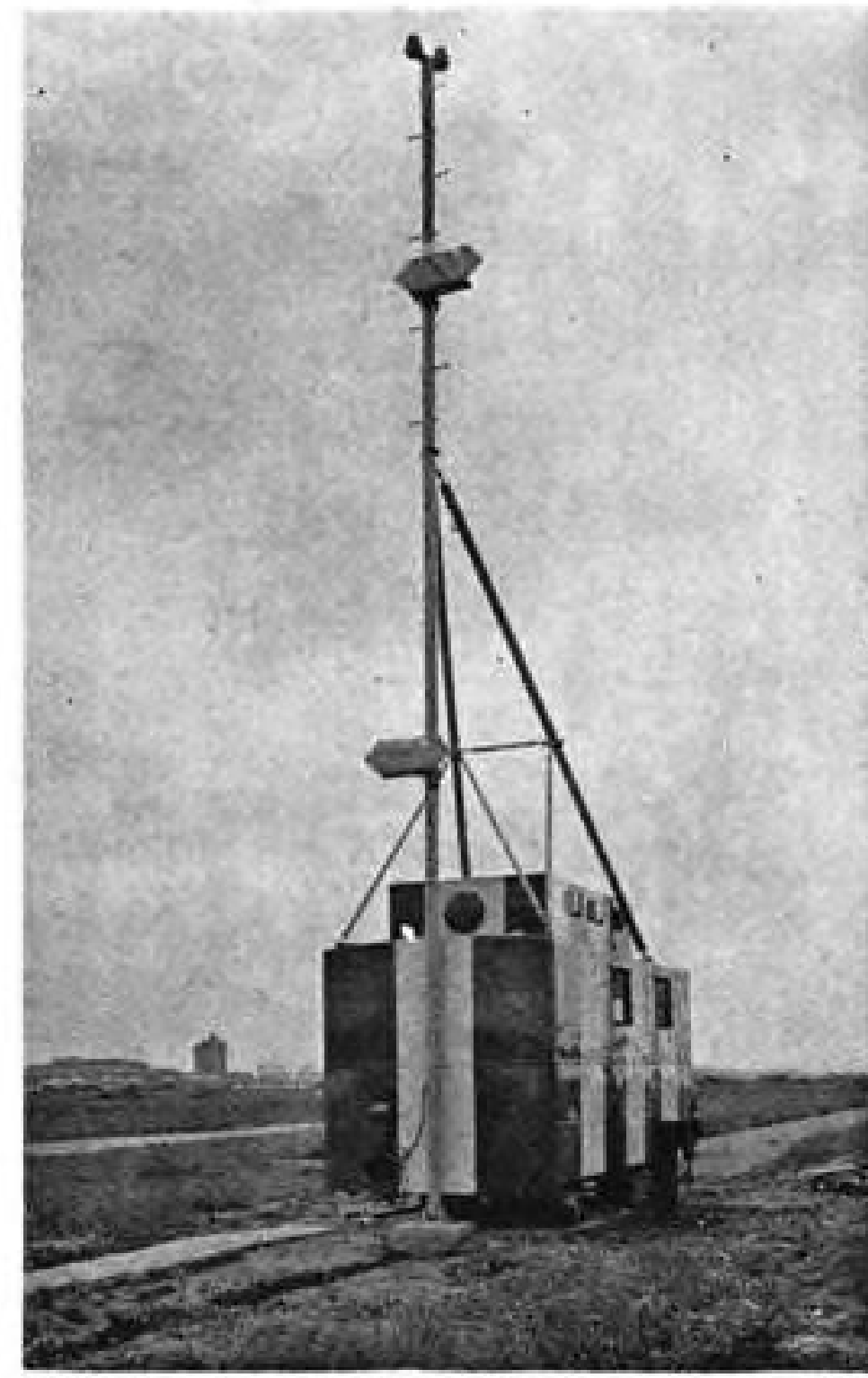
DUAL localizer antennas for STAN 7/8 ILS consist of broadside arrays of wideband dipoles 50 ft. apart (left). Glide path unit is at right.
