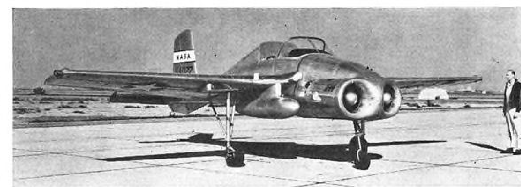
Diverted J85 thrust will power the Bell X-14 this year in a NASA test program.
