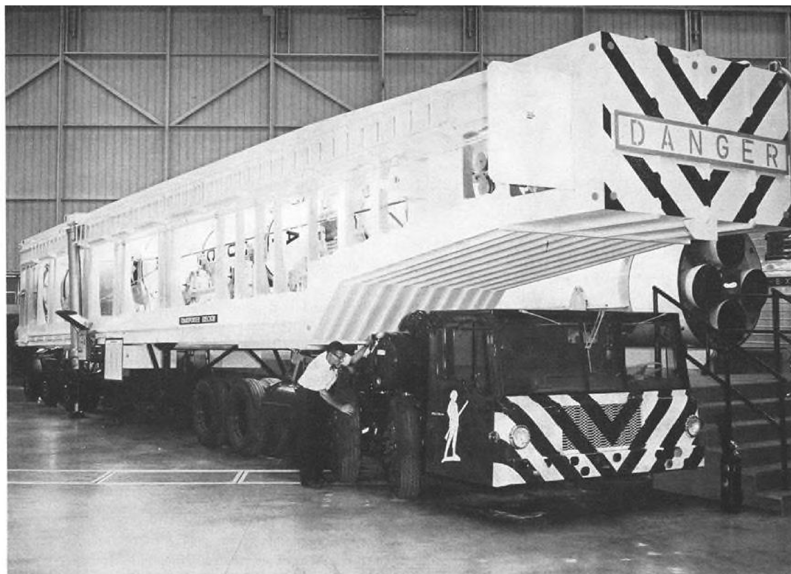
Transporter-erector for Minuteman intercontinental ballistic missile will be used to move the weapon from the assembly and recycle facility to underground silo sites. Unit also will be used to load Minuteman into transport aircraft for airlift to the sites.
