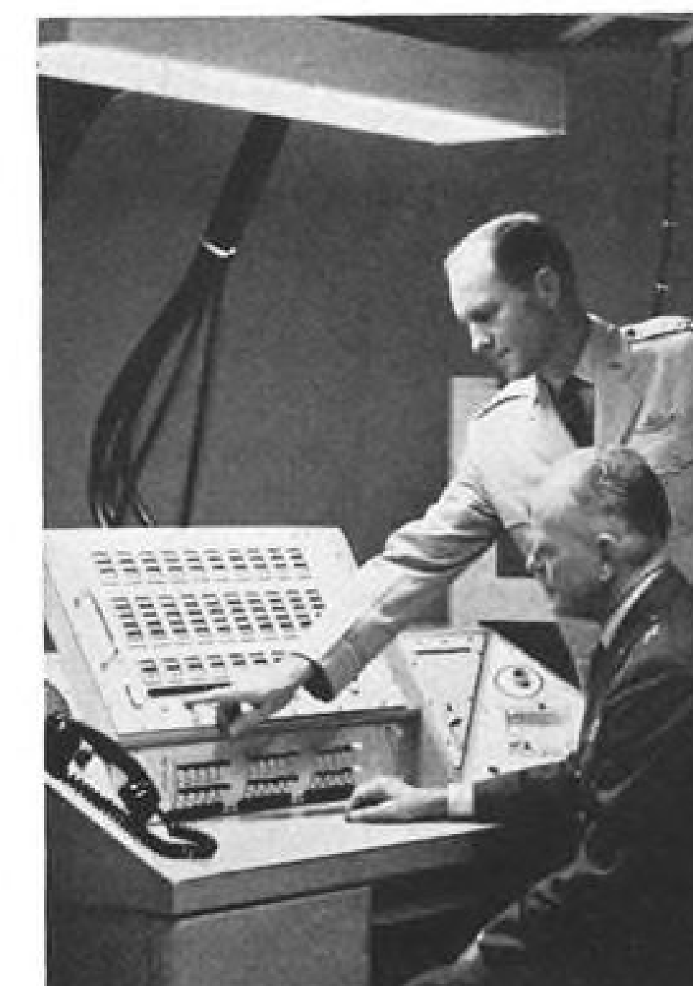
Blockhouse for Minuteman control is 29 ft. high and is part of $7 million flight test facility at Cape Canaveral. First Minuteman launch is set for December. Launch control is on first floor level; second level has a ready room, evaluation room, power supply center.
