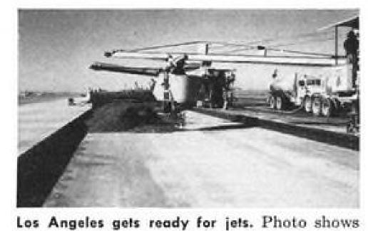
modern equipment now placing new concrete directly on the old flexible pavement of runway 25L. They're paving 1,600 feet of 25-ft. strips every working day, will take just 120 days for the whole 150-ft. x 6,150-ft. runway! Artist's sketch at top of page shows how airport will look with modern concrete runways and new futuristic-styled terminal area.
