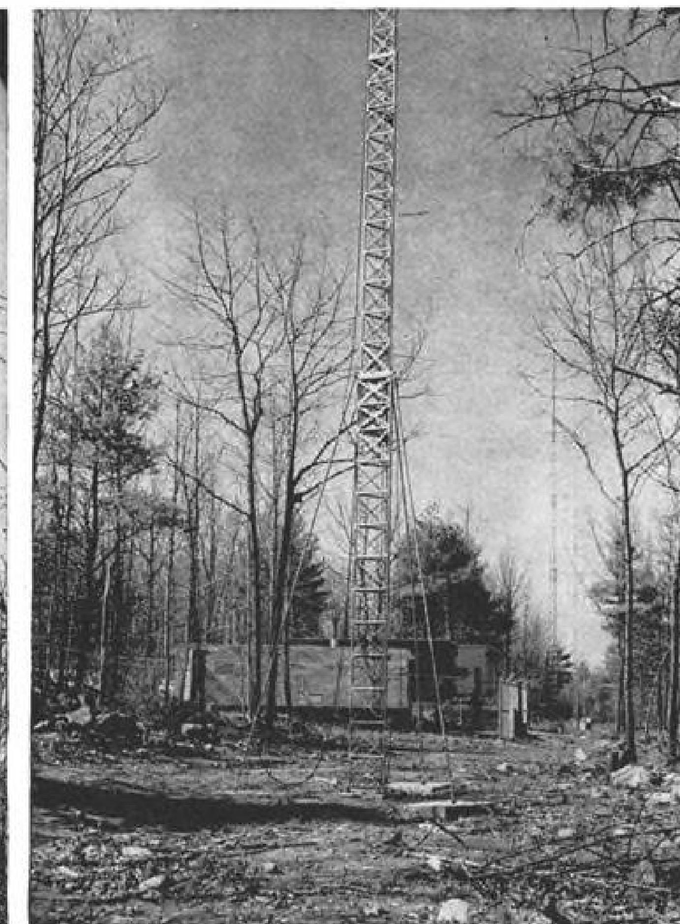
GROUND STATION ANTENNAS employed in ionospheric scatter ground-air communications tests include transmitting antenna (left), using a vertically stacked dipole which gives broad azimuth coverage but compresses radiation in vertical direction, and six receiving antennas, four of them visible in photo (right), which provide space diversity operation for receiving aircraft transmission.
