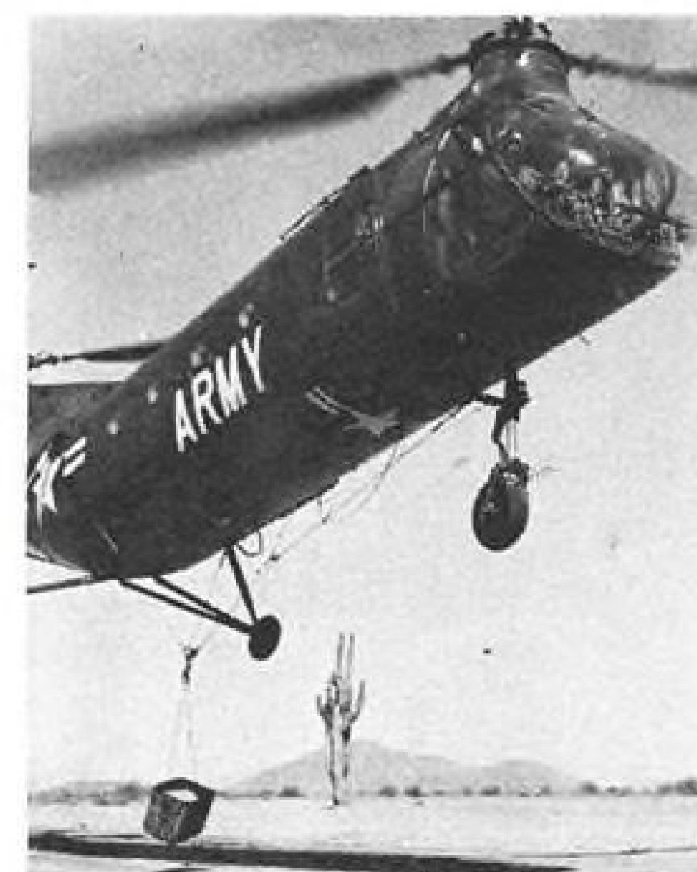
SWINGING below Army H-21 helicopter is a 600-lb. load serving as a pendulum during tests of Army-Sperry Phoenix universal flight control system in the desert near Sperry plant in Phoenix.
