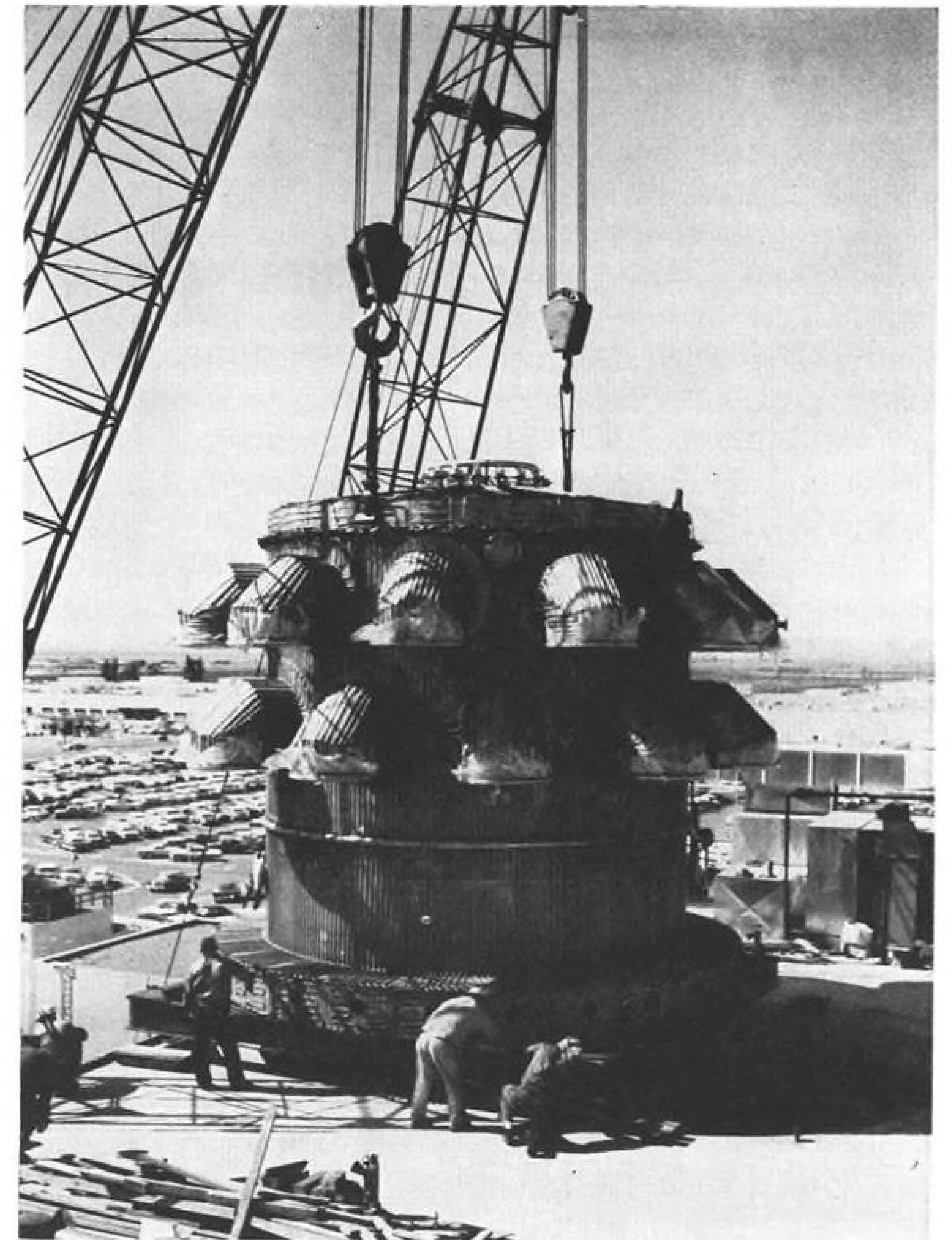
JET PROPULSION LABORATORY -designed space simulation chamber (above) is lowered into place in new Space Simulation Facility at Pasadena, Calif. Artist's conception of the new building (below) shows tower for housing artificial sunlight system. Chamber, which weighs 55 tons, rests immediately below. Protrusions on chamber are ducts which will lead to vacuum pumps. Aluminum shroud inside chamber has 200 plates to absorb heat.
