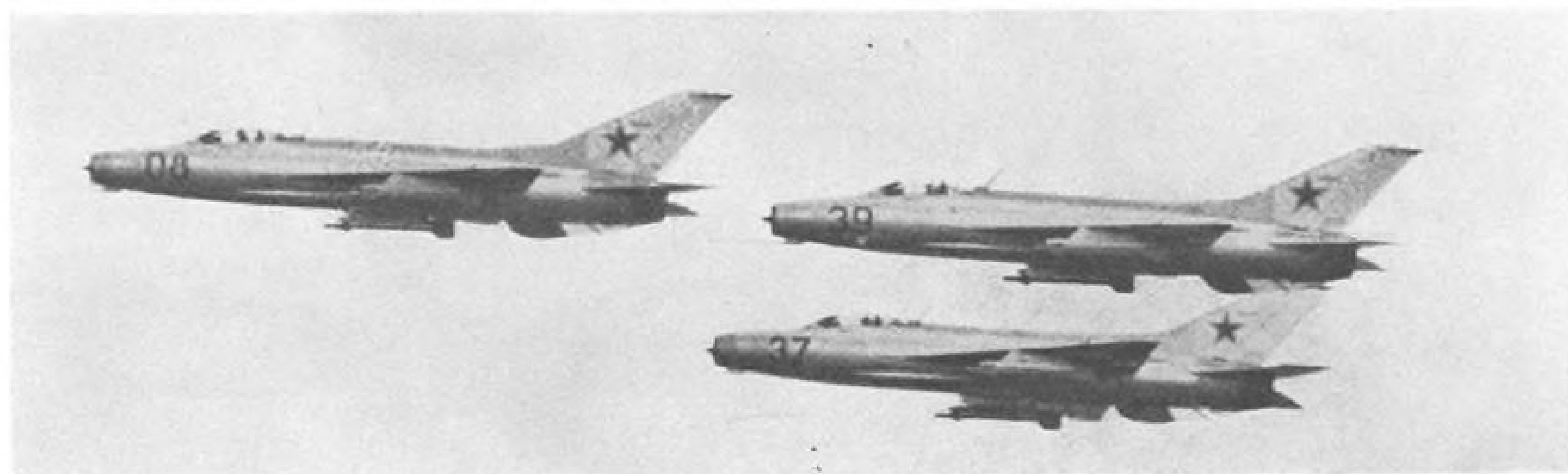
Formation of Mikoyan Fishbed Mach 2 delta-winged fighters is shown armed with a Sidewinder-type infrared missile mounted under each wing. Note large ventral fin and spiked air intake in nose. Fishbeds are in operational service with Soviet air force as well as the satellite air forces of Poland, Hungary and East Germany.
