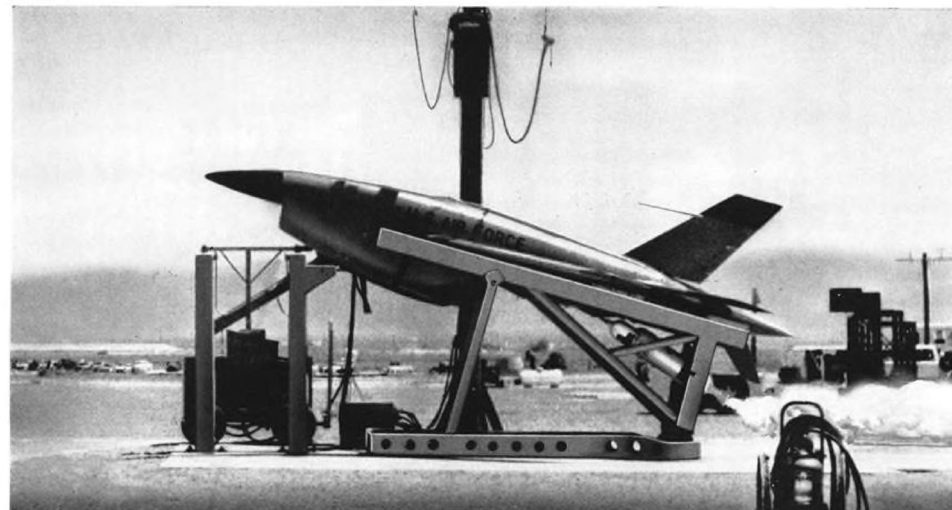
Ryan Firebee jet target being launched from a Fruehauf launcher
