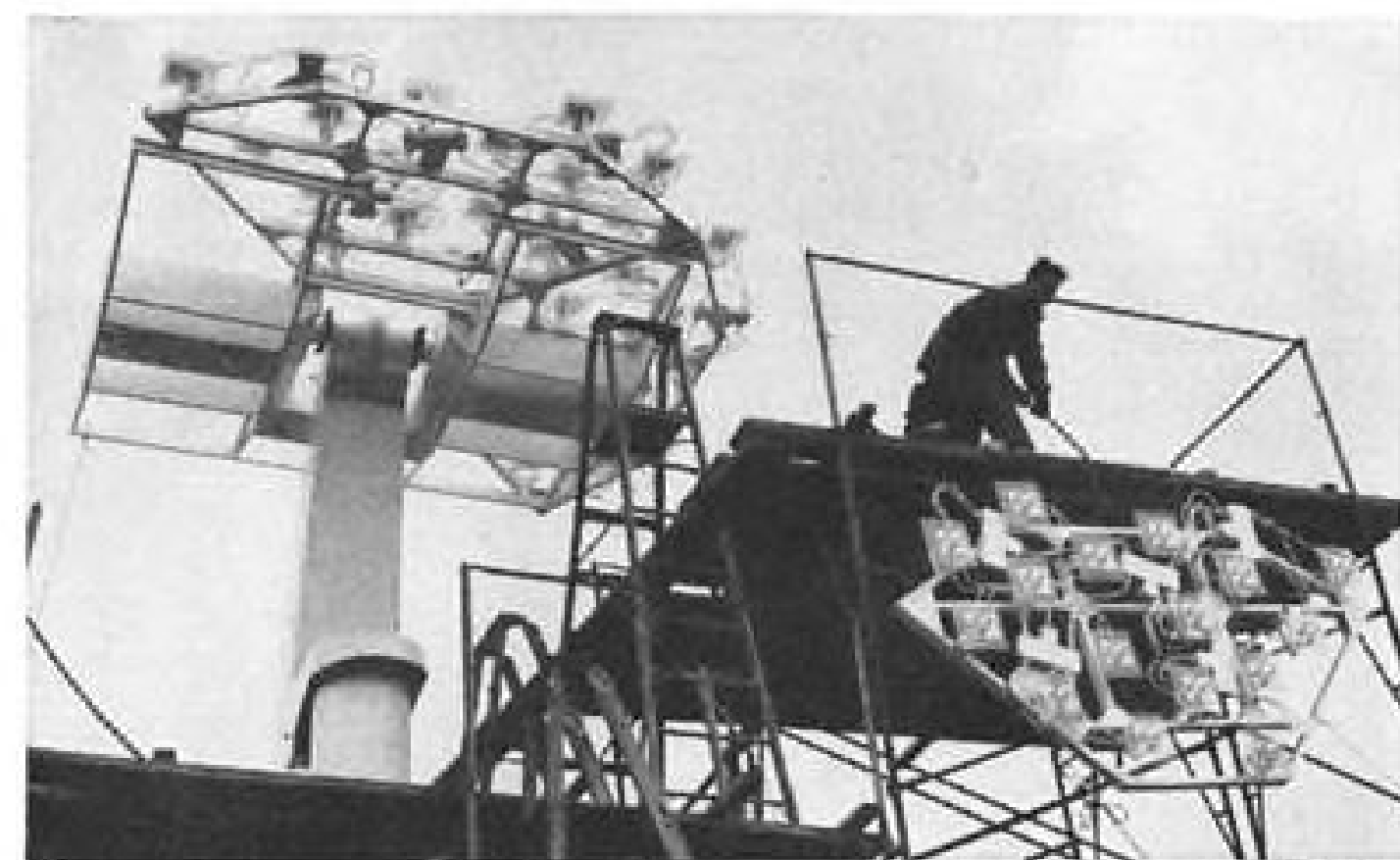
Completed quadrant elements are raised to platform for placing into position on pedestal mount.
