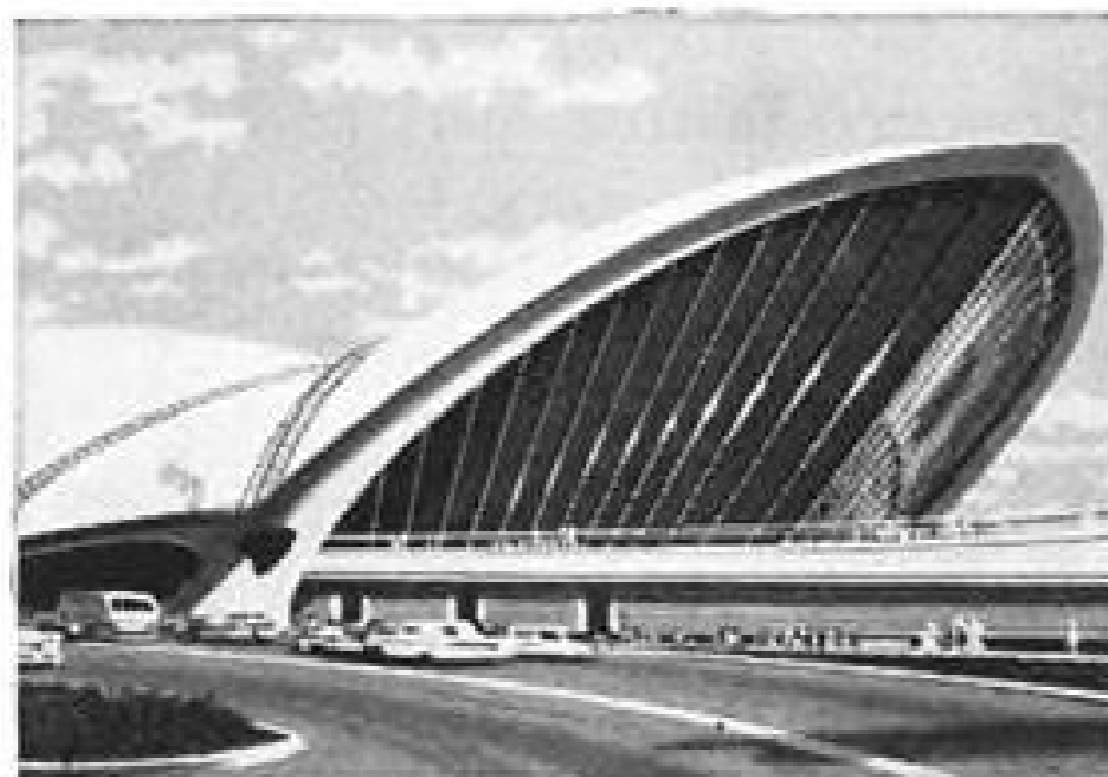
NEW YORK —this TWA terminal soon to open at the International Airport reflects the jet age in soaring concrete.
